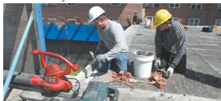
Part of the money NYCHA received from tax credits as part of the Federalization plan will be used for roof repairs.
