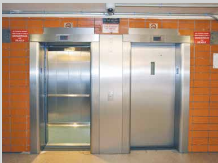
Elevator upgrades at Chelsea-Elliott Houses in Manhattan
