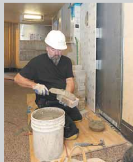
Interior refurbishing at Whitman-Ingersoll Houses in Brooklyn
