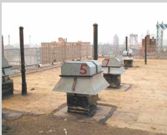
Roof repairs at Rutgers Houses in Manhattan
