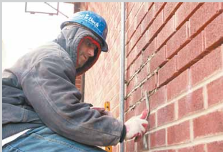
Exterior brick work at Armstrong Houses in Brooklyn
