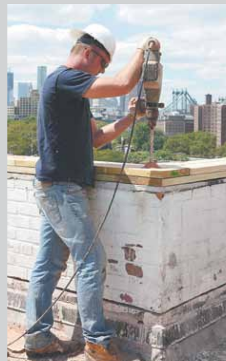
Roof repairs at Whitman-Ingersoll Houses in Brooklyn
