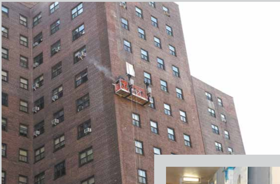
Exterior brick work at Marble Hill Houses in the Bronx
