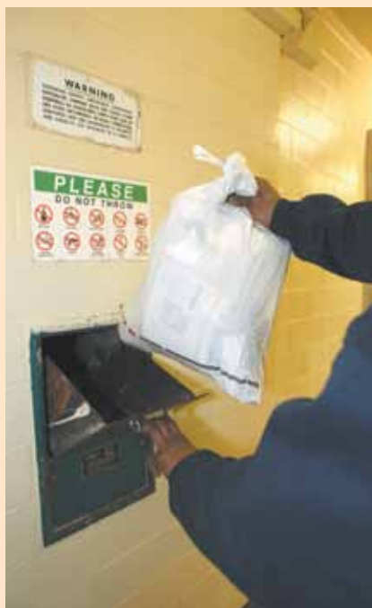
Residents should use small kitchen bags to throw garbage out in the chutes located in building hallways.
