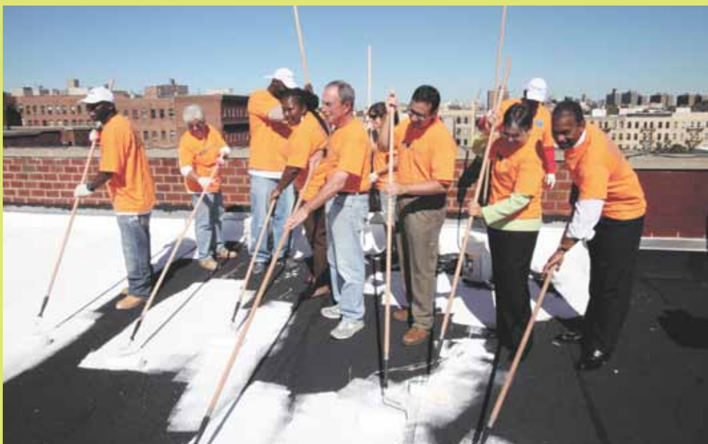
NYCHA Chairman John B. Rhea (far right) and Commissioner Margarita López (second from right) join Mayor Michael Bloomberg (center) at Betances Houses in the Bronx to coat the one millionth square foot of rooftop white by the NYC Service Cool Roof Initiative.
