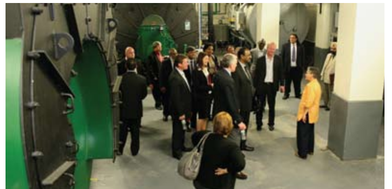
NYCHA officials show a South African delegation the new energy-efficient pass steam boilers at Castle Hill Houses in The Bronx.
