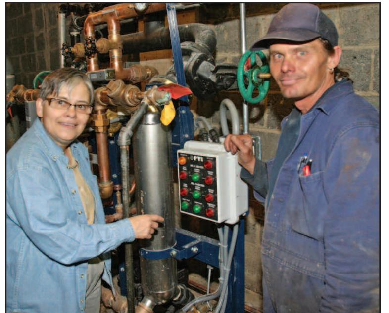
**GOING GREEN** NYCHA Board Member Margarita López and Heating Plant Technician Raymond Horn with one of the new instantaneous hot water heaters at Baruch Houses. The new heaters will significantly reduce carbon dioxide emissions while providing improved service.
