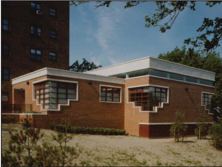
St. Mary's Park Community Center in the South Bronx.
