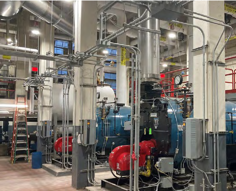
CENTRAL HEAT PUMP DOMESTIC HOT WATER HEATER
