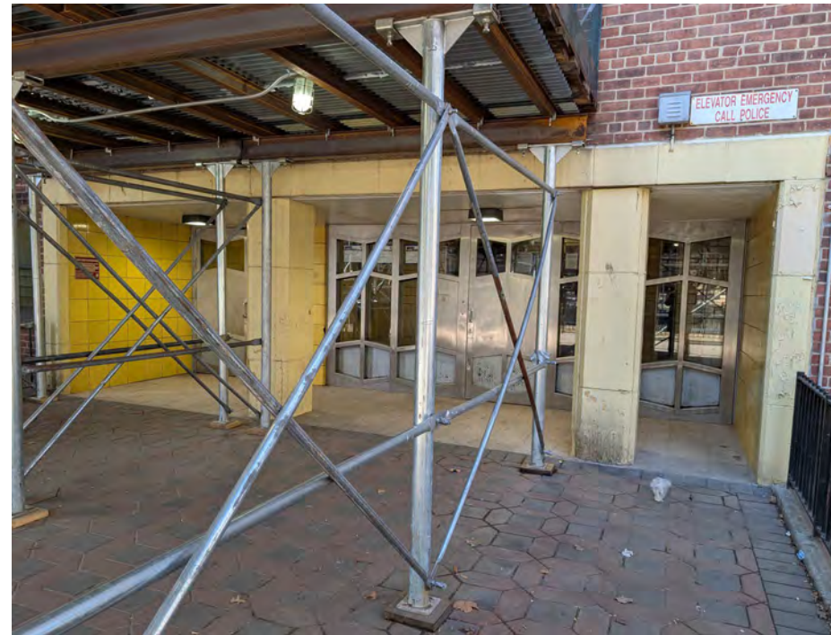
A typical building entrance
