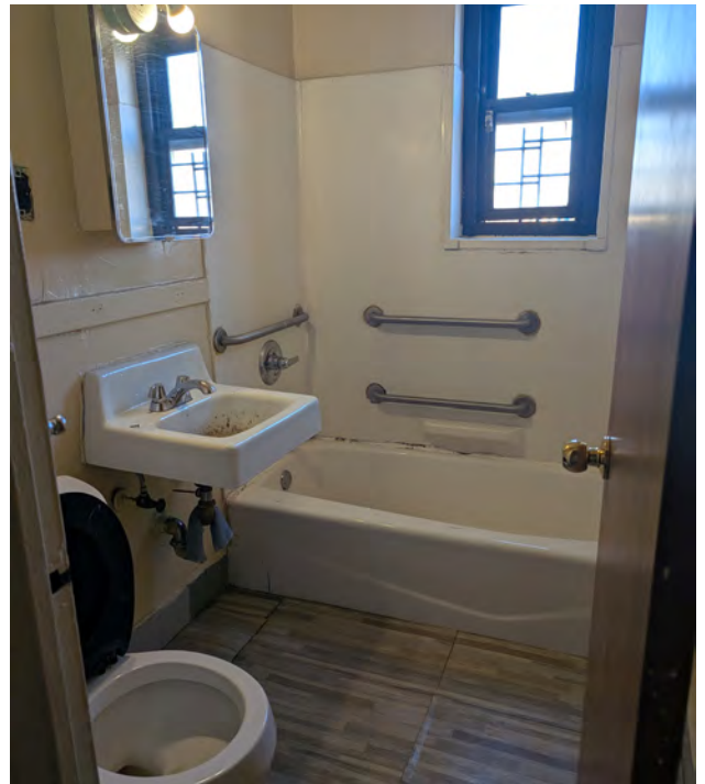
EXISTING BATHROOMS BAÑOS EXISTENTES HAITIAN CREOLE
