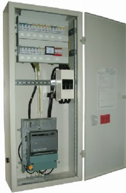
Water tight seals on electrical panels
