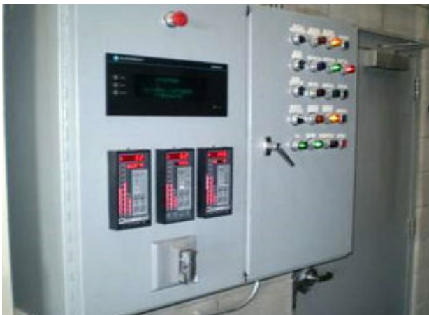
Boiler Control Panels
