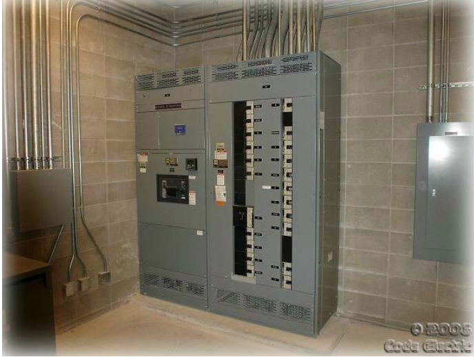
Elevated switchgear
