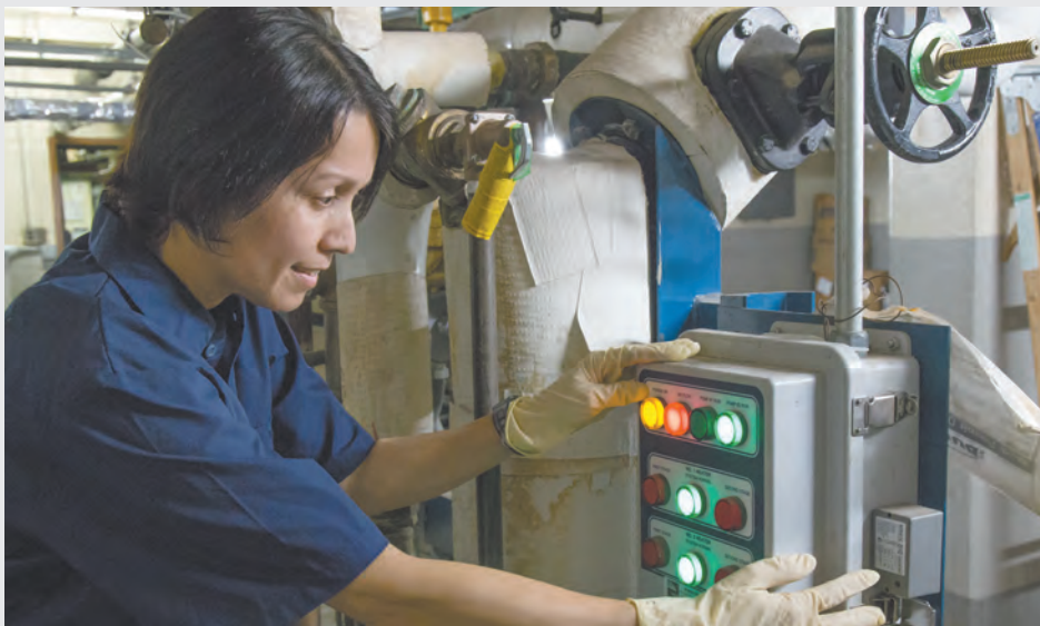
Lillian Hernandez, a Heating Plant Technician, conducts a variety of safety tests on boilers at Whitman Houses to make sure they’re working properly so that residents have hot water and are warm when it’s cold outside.
