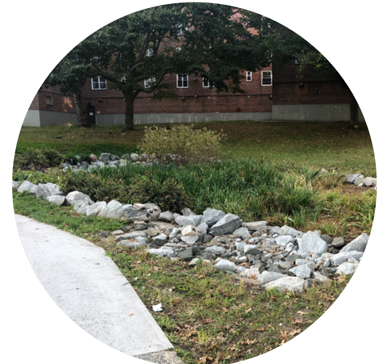
Green infrastructure installation at Edenwald Houses.
