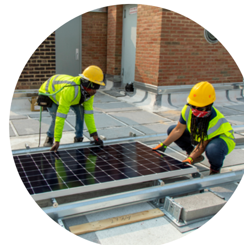
Solar panel being installed at Queensbridge Houses.
