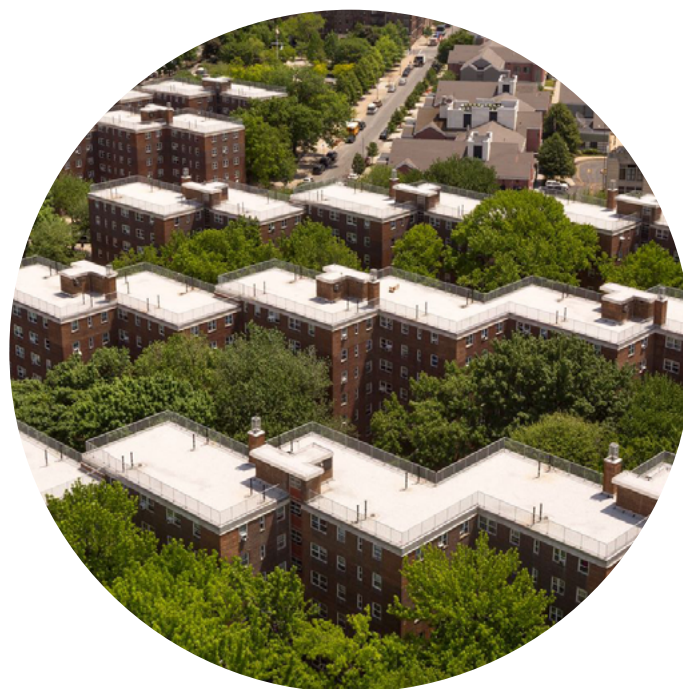
Kingsborough Houses underwent exterior renovations which included façade repairs, asbestos abatement, brick replacement, parapet replacement and reroofing.
