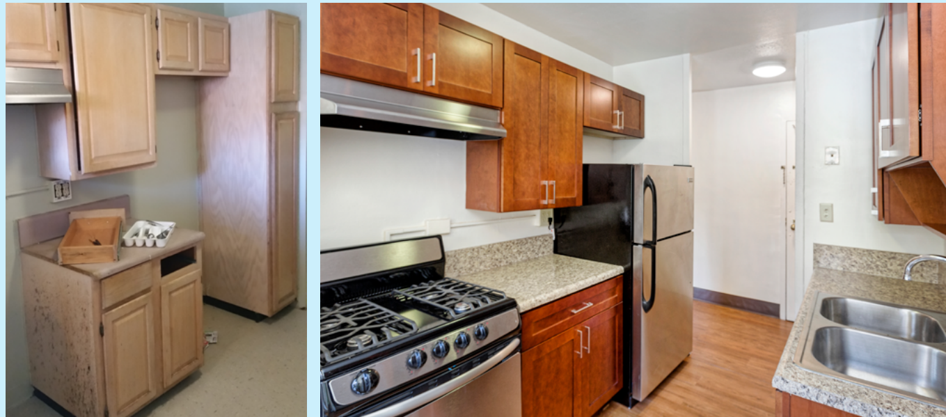
On the left, Ocean Bay apartment before PACT transition and renovations completed. On the right, Ocean Bay apartment after PACT renovations completed in 2019.
