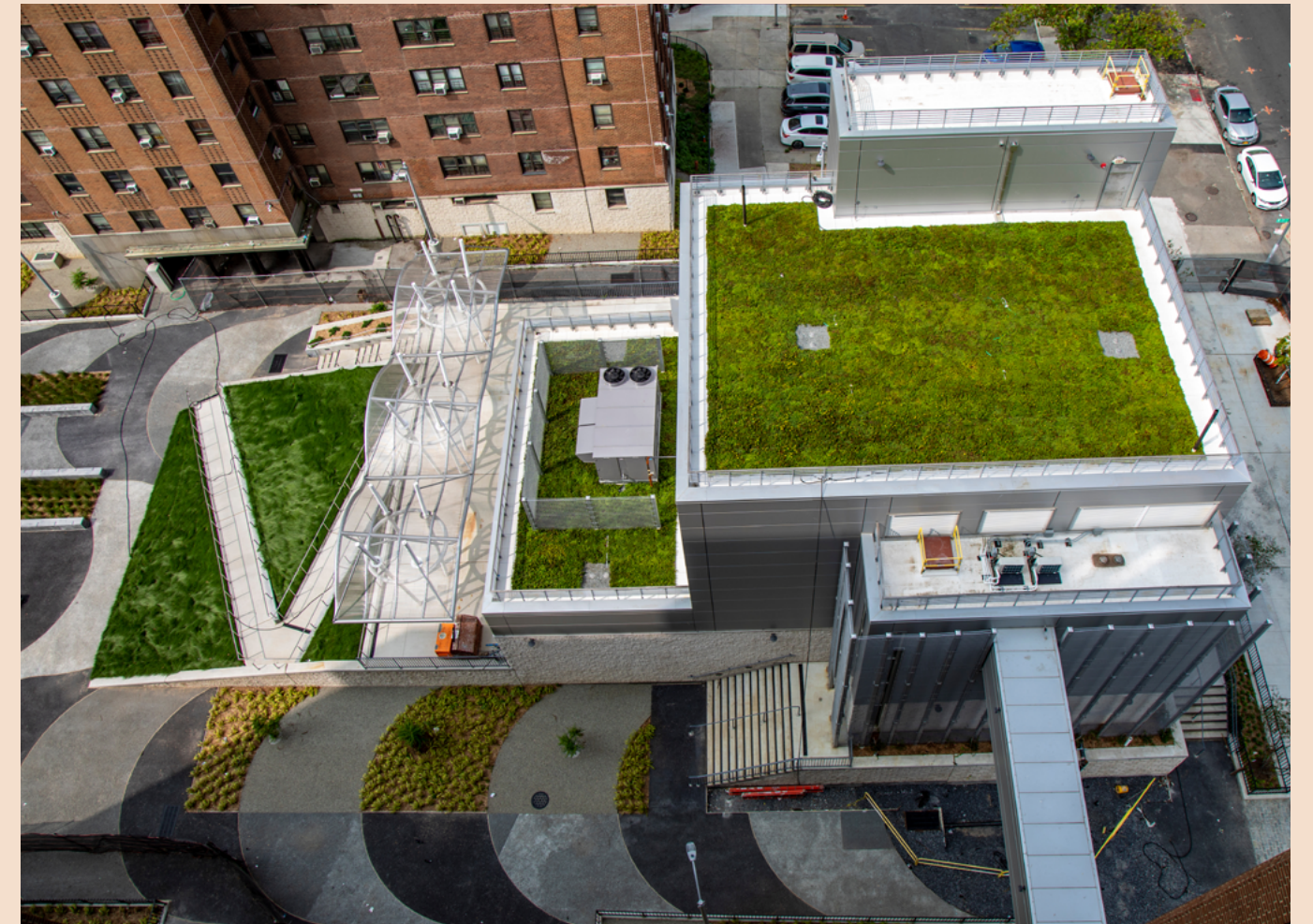
Aerial view of green roof
