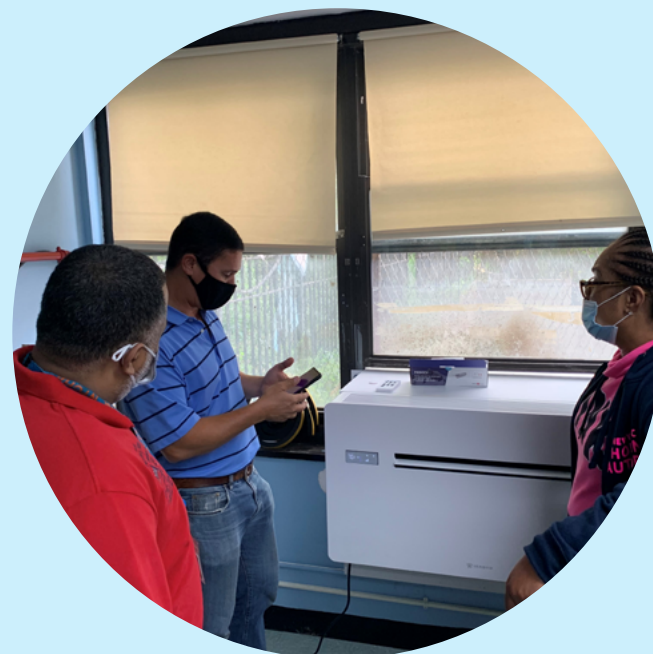
A prototype window-mounted heat pump is installed at Fort Independence.
