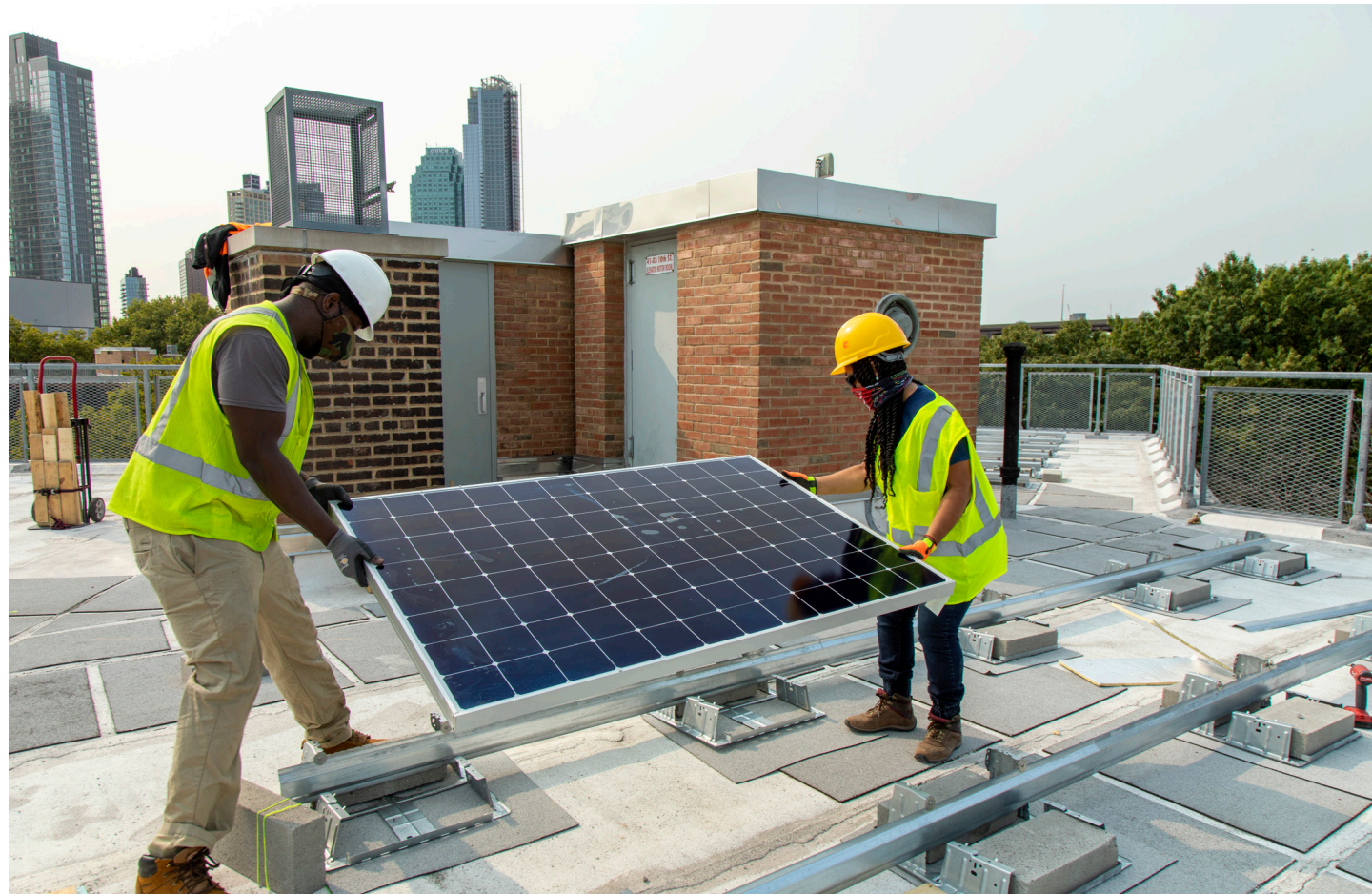
While NYCHA's community solar program at Queensbridge are not subject to Section 3, it is built into the solicitation process and lease agreements; that led to resident involvement in hiring and training residents for solar installation
