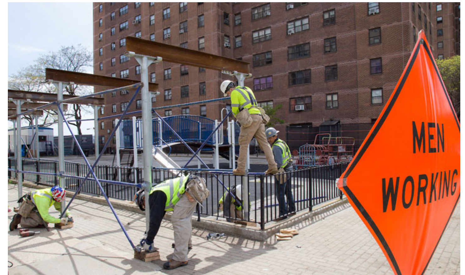
Construction groundbreaking at Coney Island Houses
