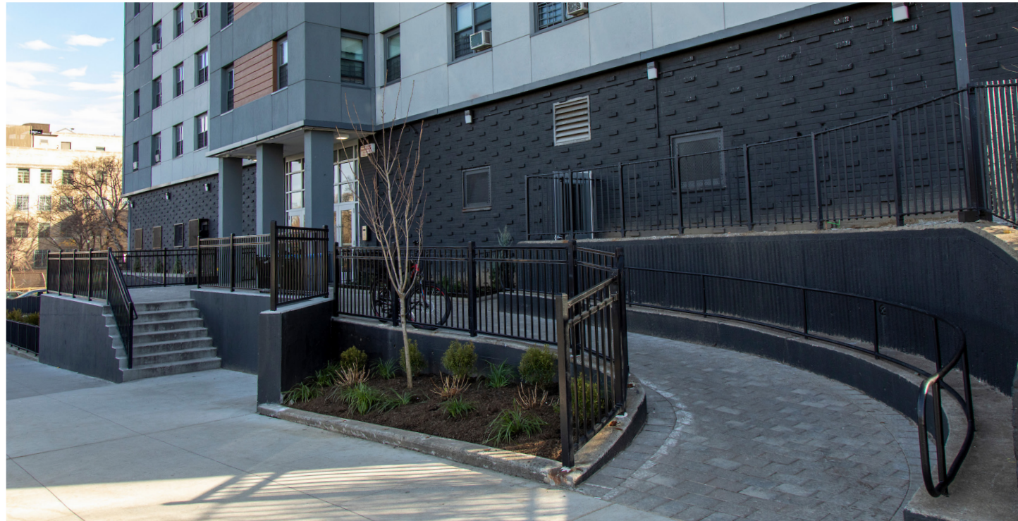
Accessible entryways at converted PACT development, Baychester Houses
