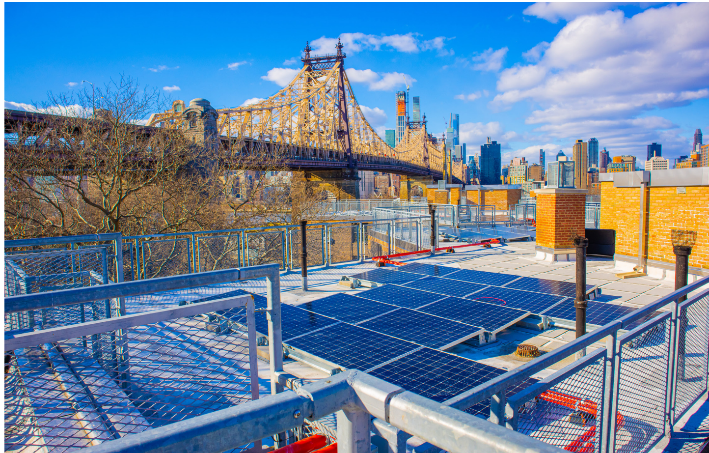
Queensbridge Houses community shared solar installation
