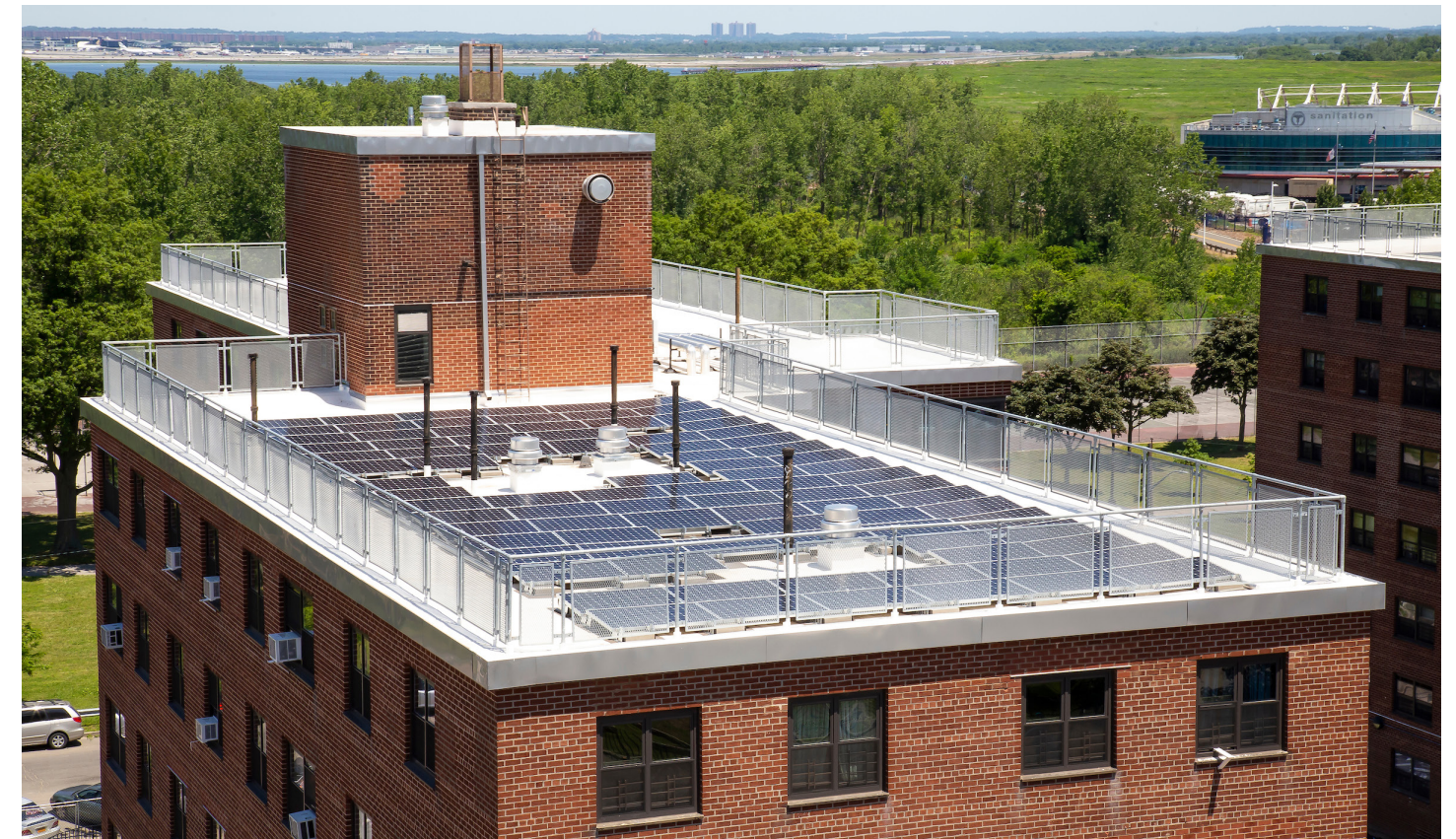
Rooftop solar installations at converted PACT development, Ocean Bay Houses
