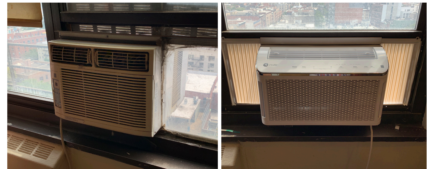
Before-after images of Smart AC installation at Meltzer Towers
