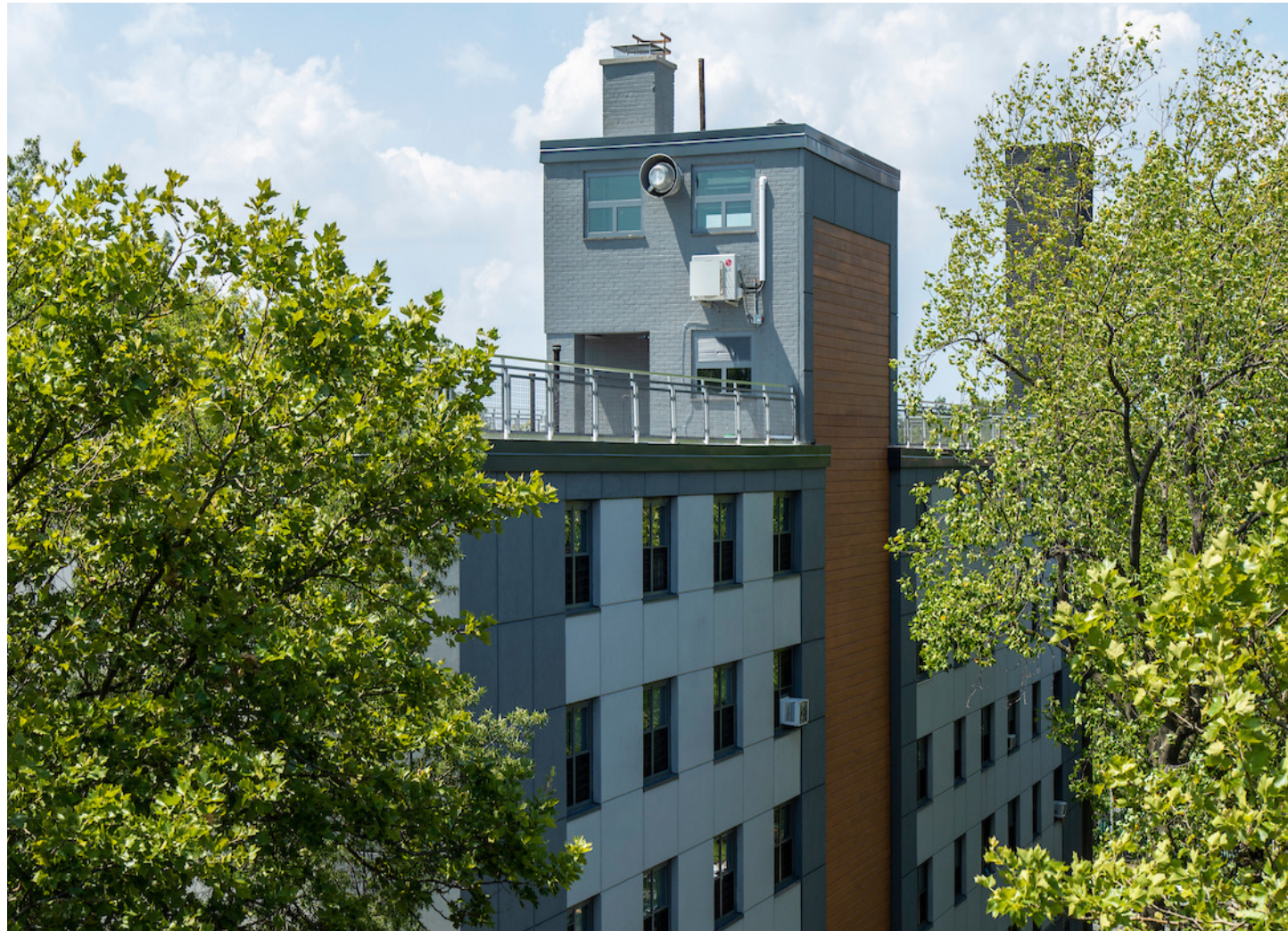
Renovated facade and windows at converted PACT development, Baychester Houses
