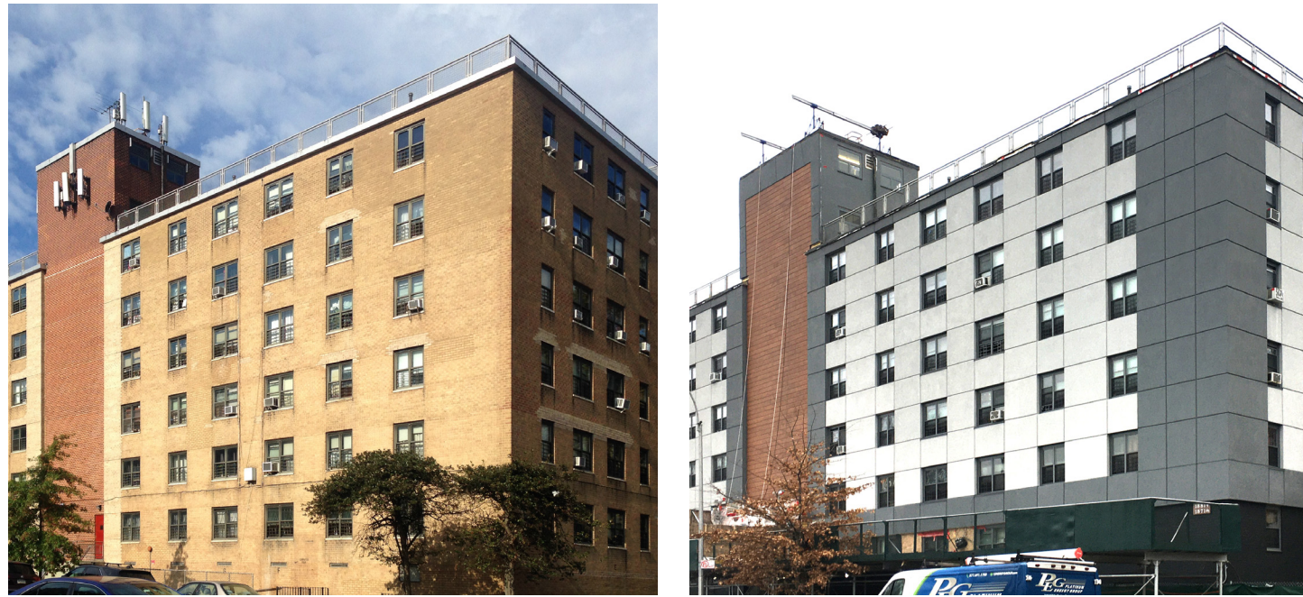
Before-after imagery of renovations at converted PACT development, Baychester Houses
