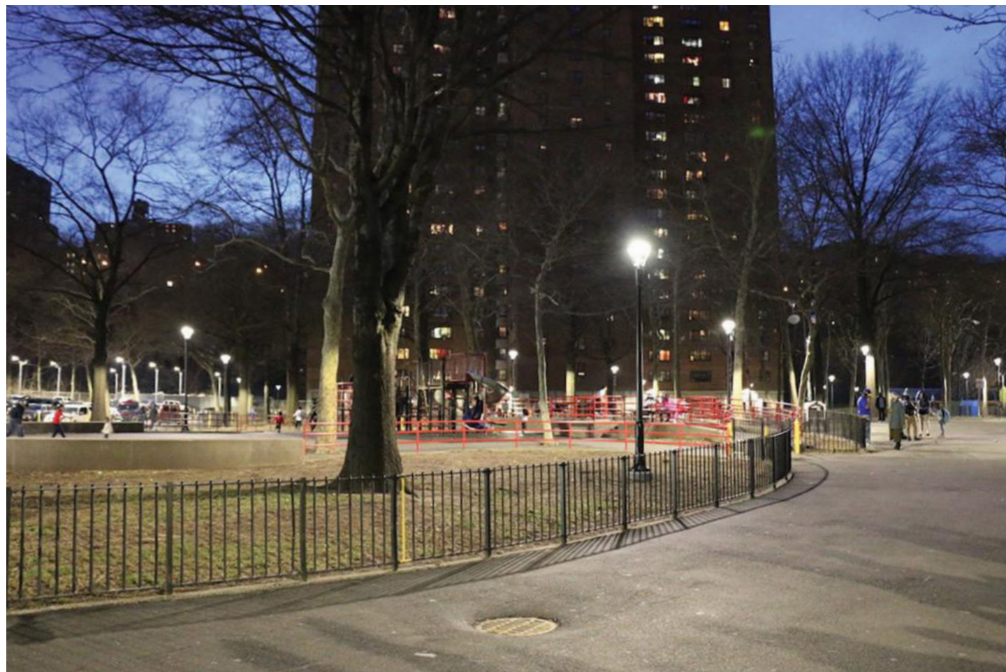
Upgraded exterior lighting at Polo Grounds Towers
