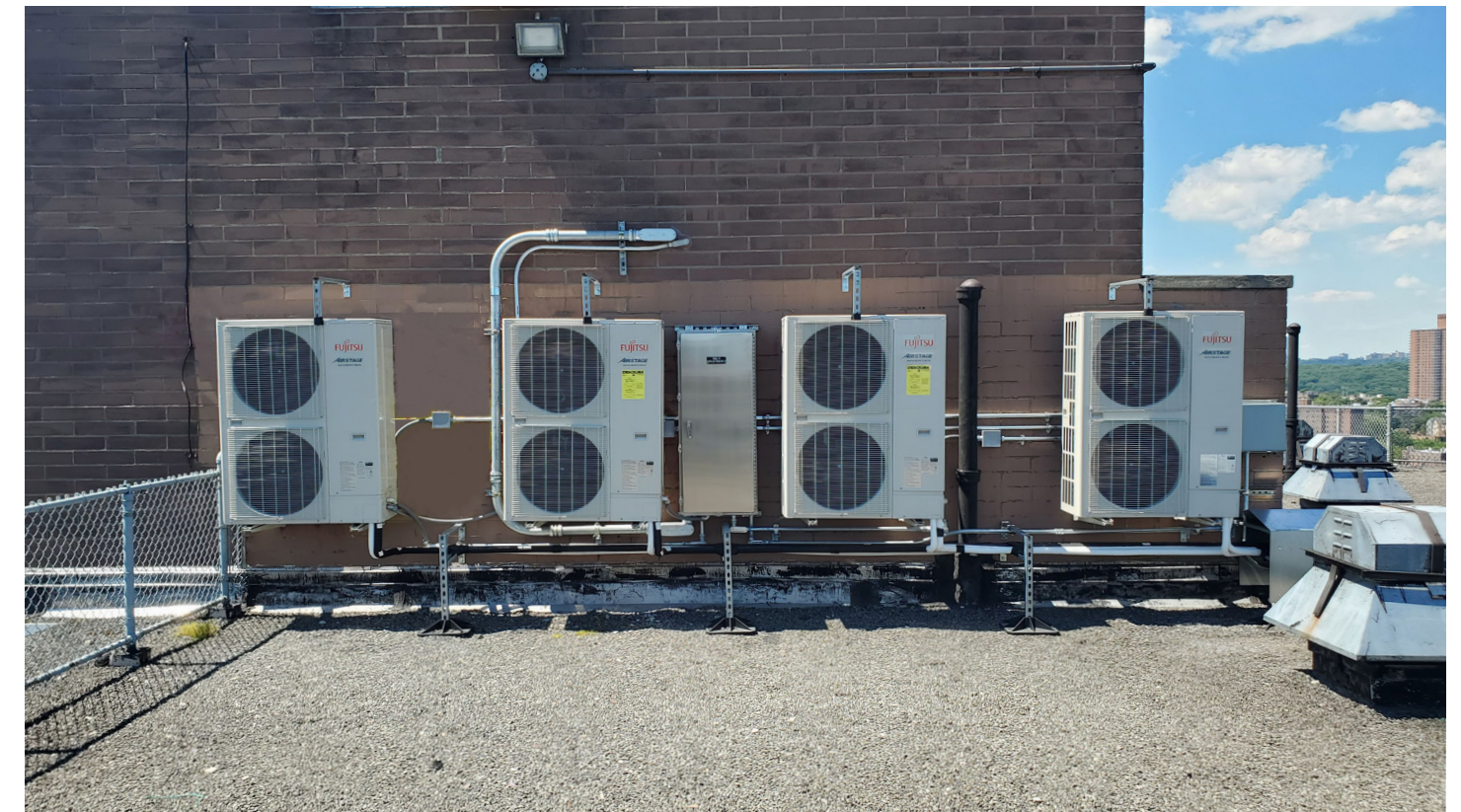
Outdoor units of heat pumps systems at Fort Independence
