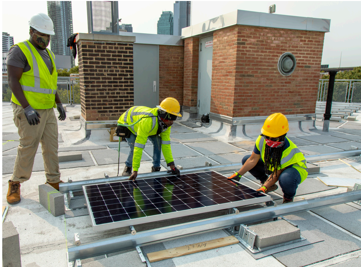
Queensbridge Houses community shared solar installation
