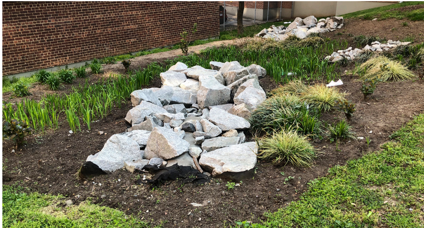
Green infrastructure installation at Edenwald Houses
