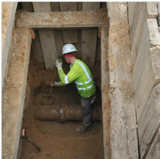
Photos from Mariner's Harbor Sewer Line Replacement circa 2023. From left to right: shoring and bracing for soil stabilization, pipe replacement, re-pavement.
