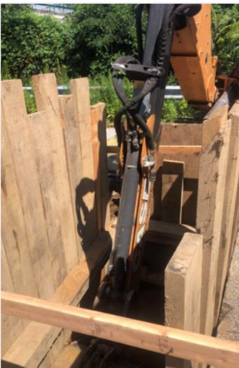
Photos from Mariner's Harbor Sewer Line Replacement circa 2023. From left to right: shoring and bracing for soil stabilization, pipe replacement, re-pavement.
