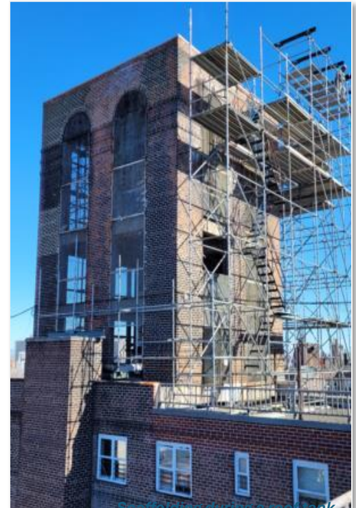
Scaffolding during a roof tank replacement at Patterson Houses
