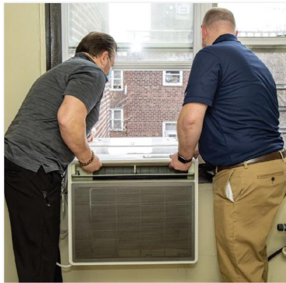
Triple-pane casement windows with new cold climate window heat pumps at Woodside Houses developed through the Clean Heat for All program
