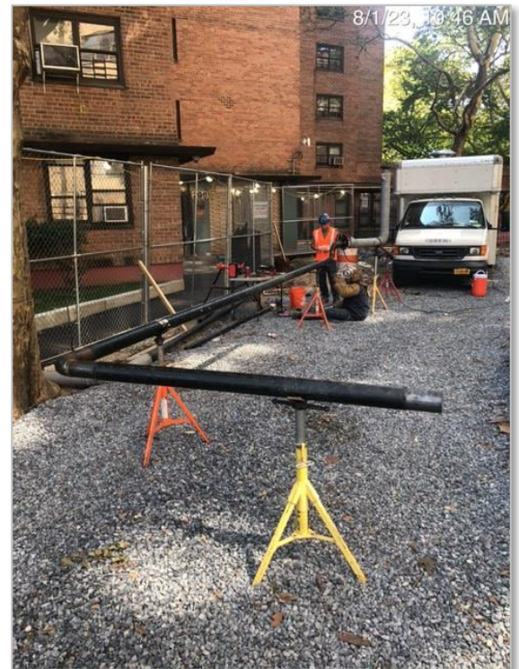
Baruch Houses, installation of a new gas line.
