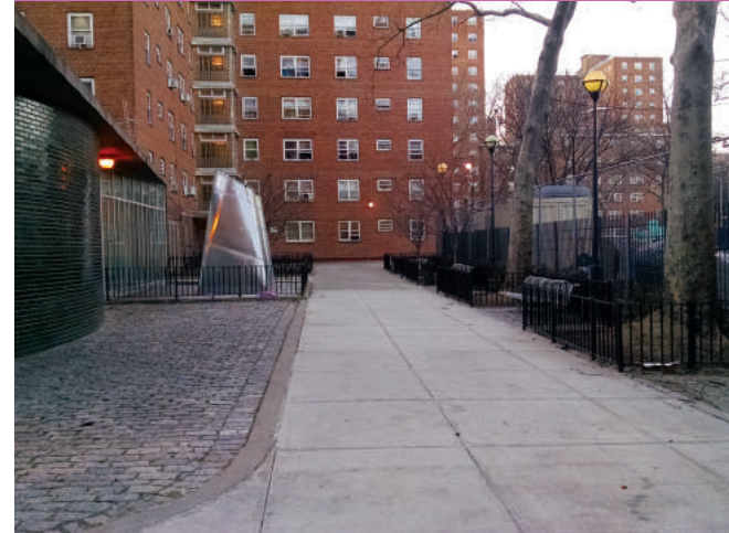
Pathway at Johnson House, made of concrete and Belgian blocks, which are easy to replace.
