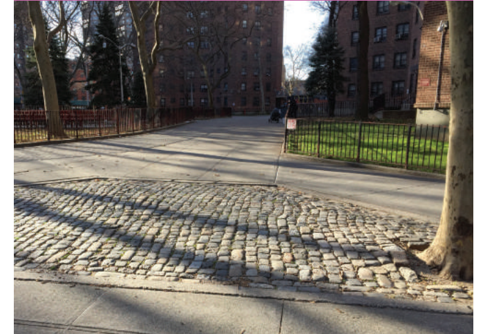
Pavement at Taft Houses, where material and pattern changes facilitates people's sense of orientation.
