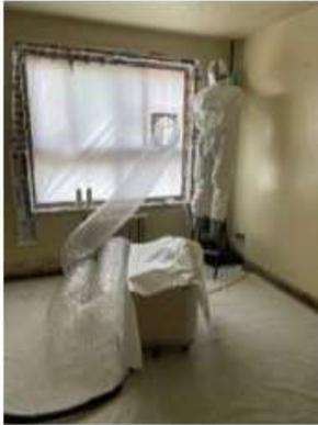
Abatement worker applying peel-away. Mechanical ventilation system in use. (Building 2 – 210K W 153<sup>rd</sup> St, Apt 3A)
