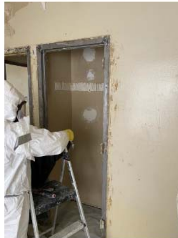
Chemical stripper/peel away (Building 3, 191V)
