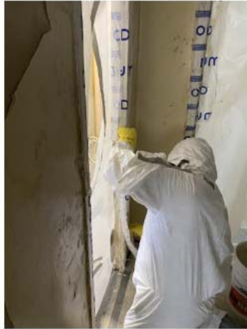
Chemical stripper/peel away (Building 3, 211G)
