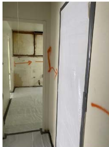
Critical Barrier (Building 5 SH32, Apt 1B)
