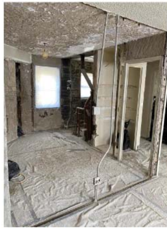
Abated walls and ceiling (Building 5 SH30, Apt 4C)
