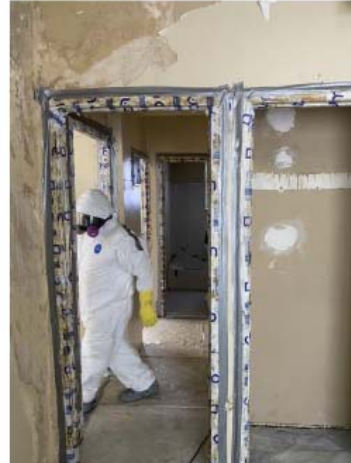
Chemical stripper/peel away (Building 3, 211G)
