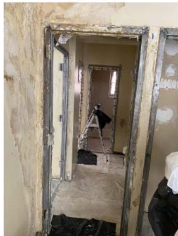
Chemical stripper/peel away (Building 7, 191V)
