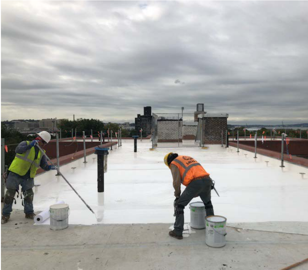
Ongoing Work Red Hook East Buildings: 1E, 14E
