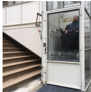
Installing a lift
