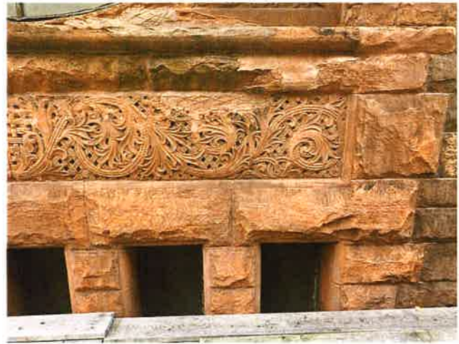
South Church – Spalled stone at ridge beam. South Church - Spalled stone and patches.
