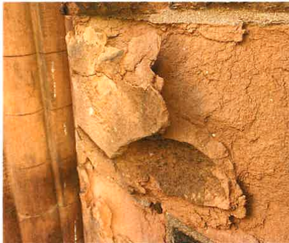
South Tower – Spalled Stone
