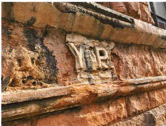
West Church - Spalled stone and patches.
