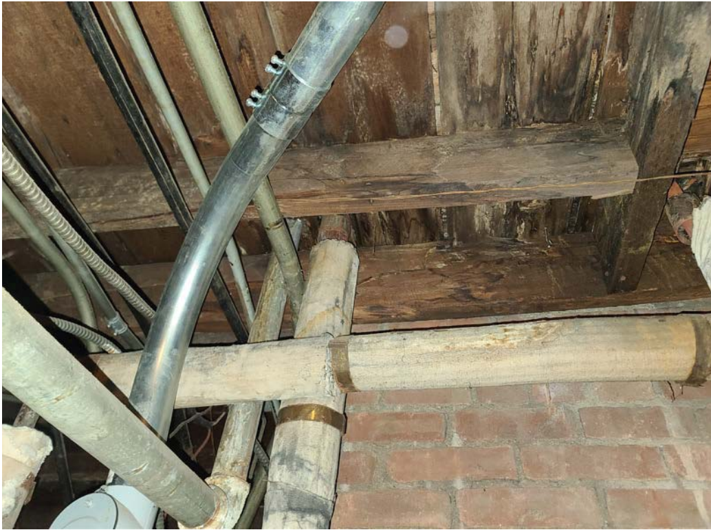
PHOTO 7: DAMAGED WOOD BEAM AND JOISTS UNDER ENTRY VESTIBULE
