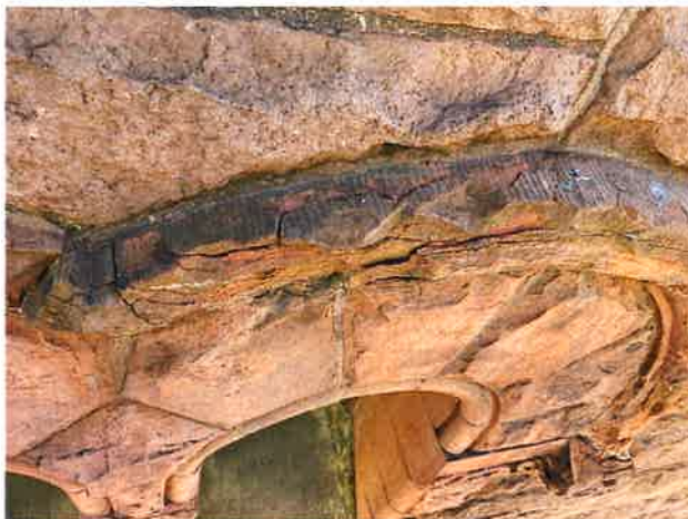
West Church – Spalled stone at window. West Church – Stained glass window compromised.
