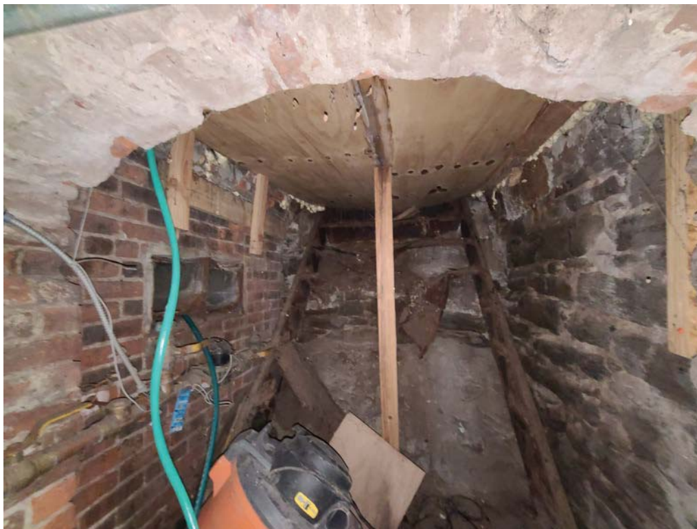
PHOTO 8: INADEQUATE SIDEWALK VAULT COVER SUPPORT
