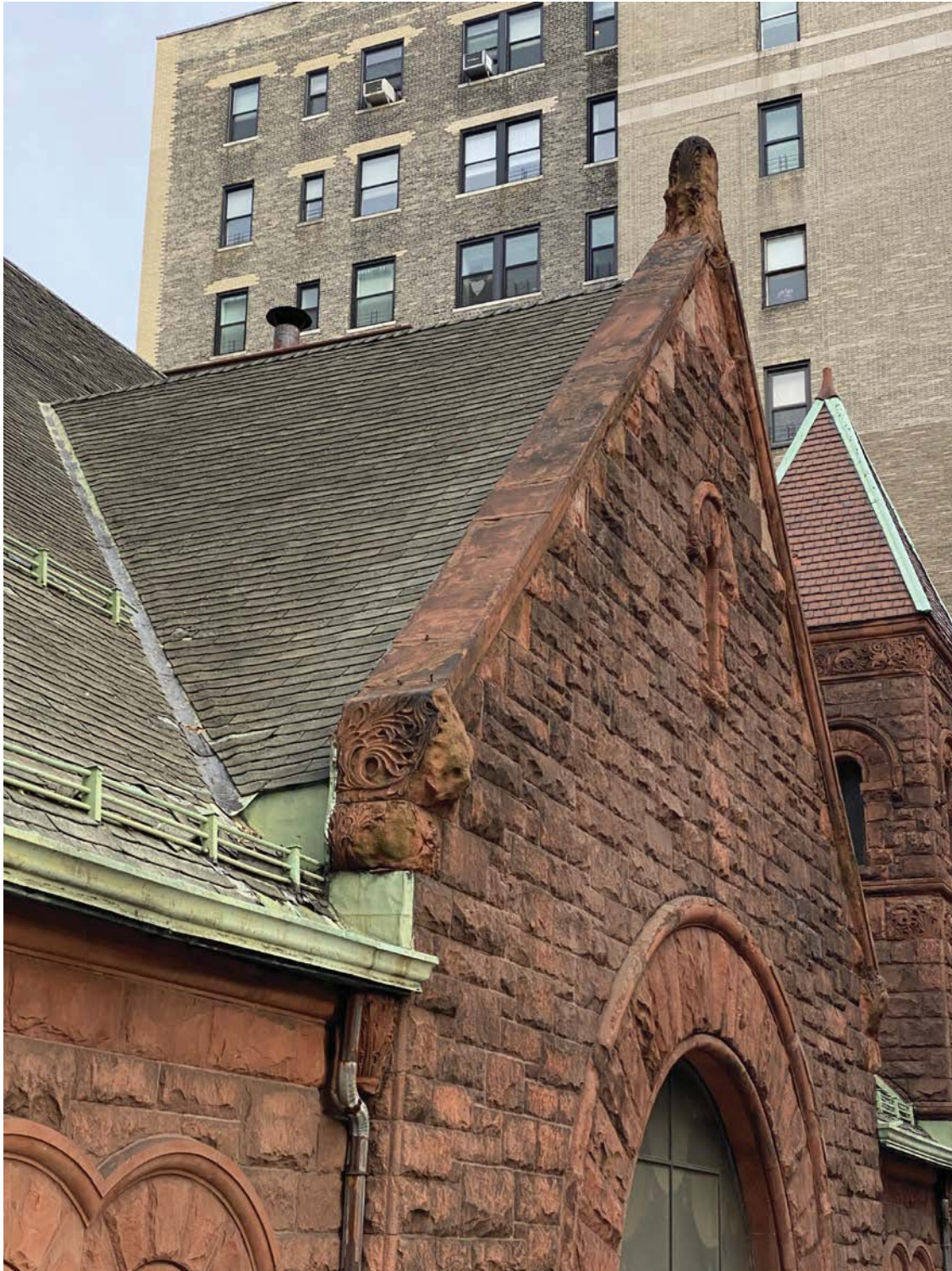
PHOTO 1: UNBRACED SECTION OF WALL
