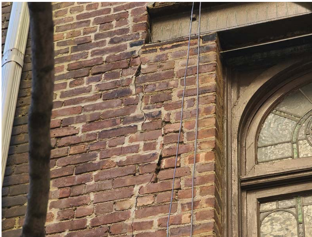
PHOTO 4: CRACKS IN BRICK EXTERIOR BEARING WALL
