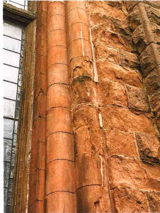
East Tower – Spalled Stones
