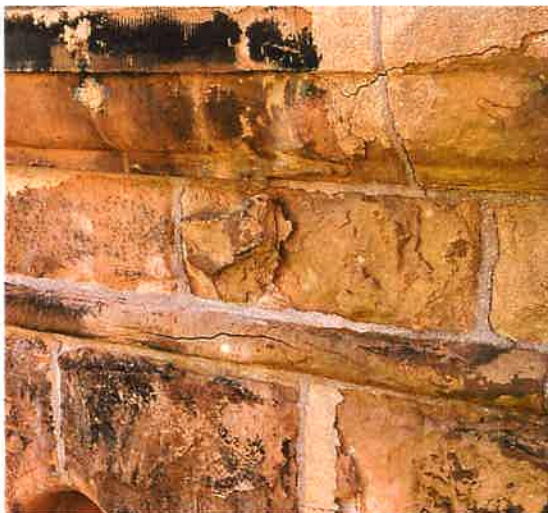
West Tower – Spalled Stone and Patches
