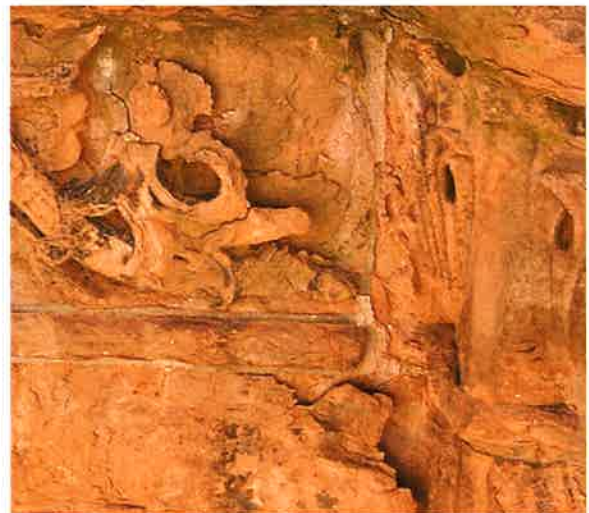
West Tower- Spalled and Deteriorated Stone
