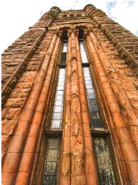
East Tower – Spalled Column Stones
