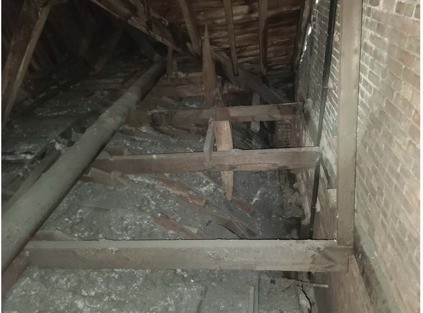
PHOTO 2: DETACHED WOOD FRAMING ADJACENT TO WALL
