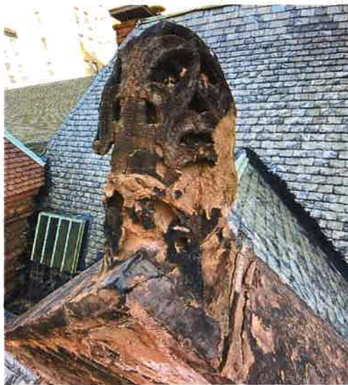
Stone is cracked and spalled
