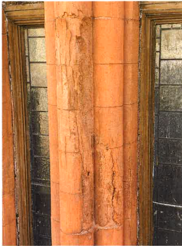
West Tower – Cracked and Spalled Column Stones
