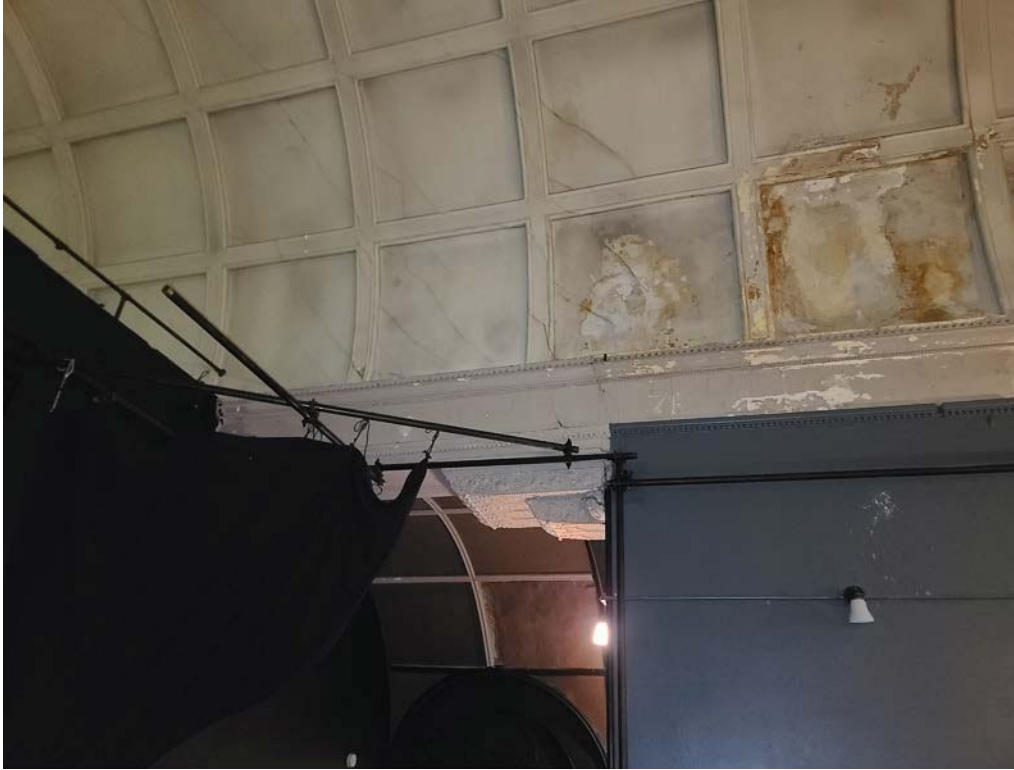
PHOTO 5: CRACKS AND DISCOLORATION NEAR BEARING END OF WOOD TRUSS
