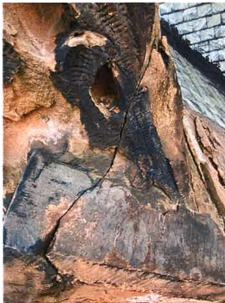
Closeup of crack that goes completely through the stone.
