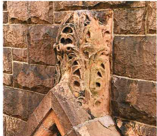
Stone Tower – Spalled Stone
