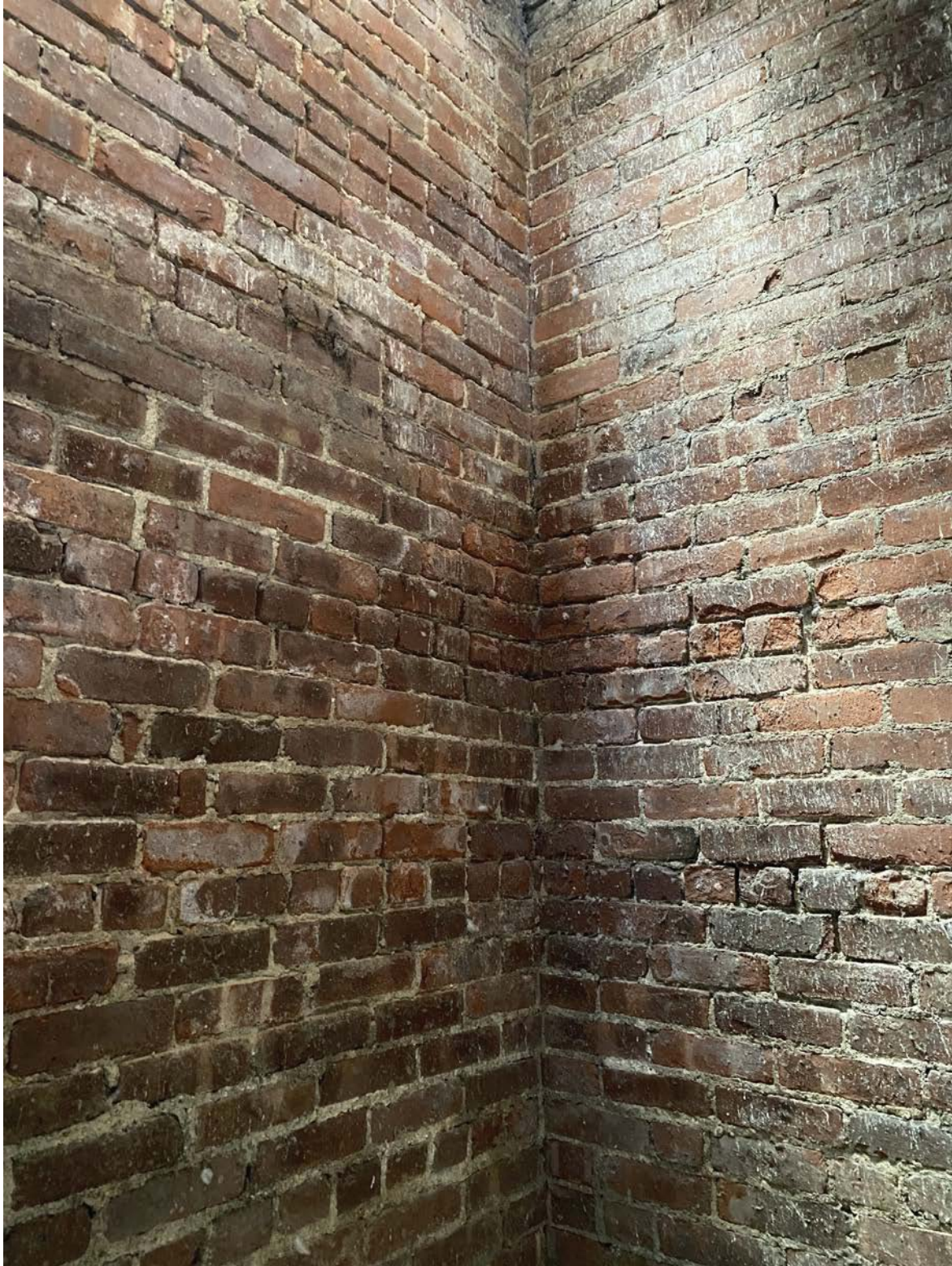
PHOTO 11: BELL TOWER BRICK REQUIRES POINTING
