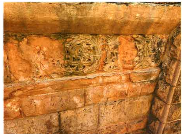
West Church - Spalled and detached stone.
