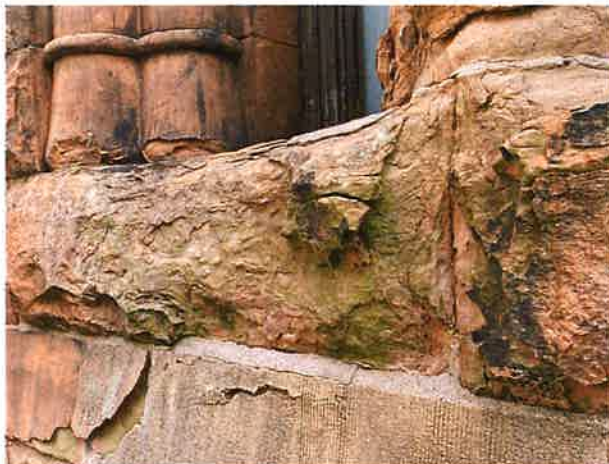
South Tower - Spall Stone at Sill
