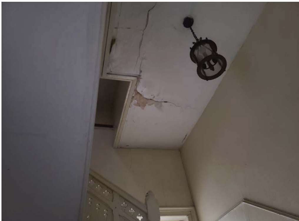
PHOTO 10: CRACKS AT STAIR LANDING UNDERSIDE
