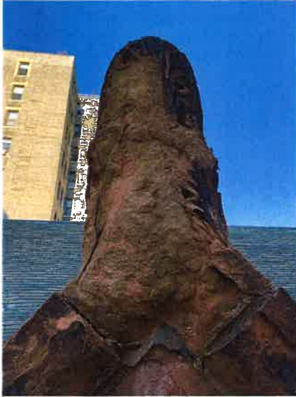
South Church – Spalled stone at ridge beam. South Church - Spalled stone and patches.
