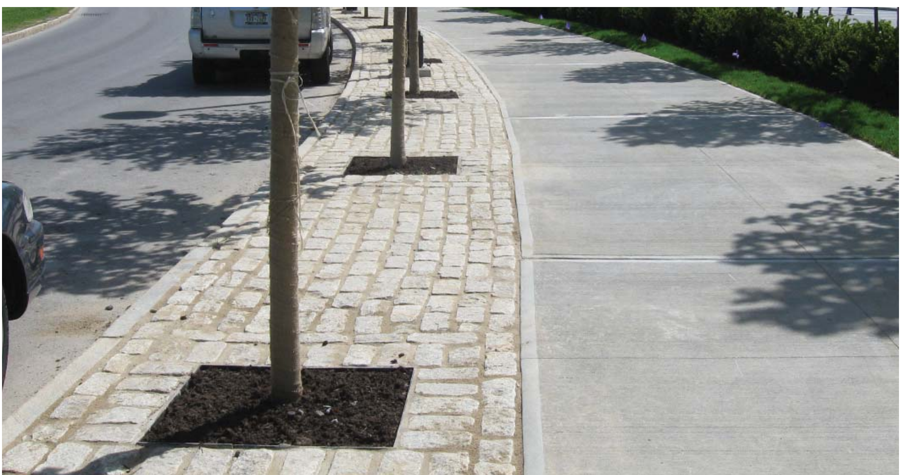
PAVING AT STREETSCAPE GRANITE COBBLE AT STREET TREES + POURED IN PLACE CONCRETE SIDEWALK
