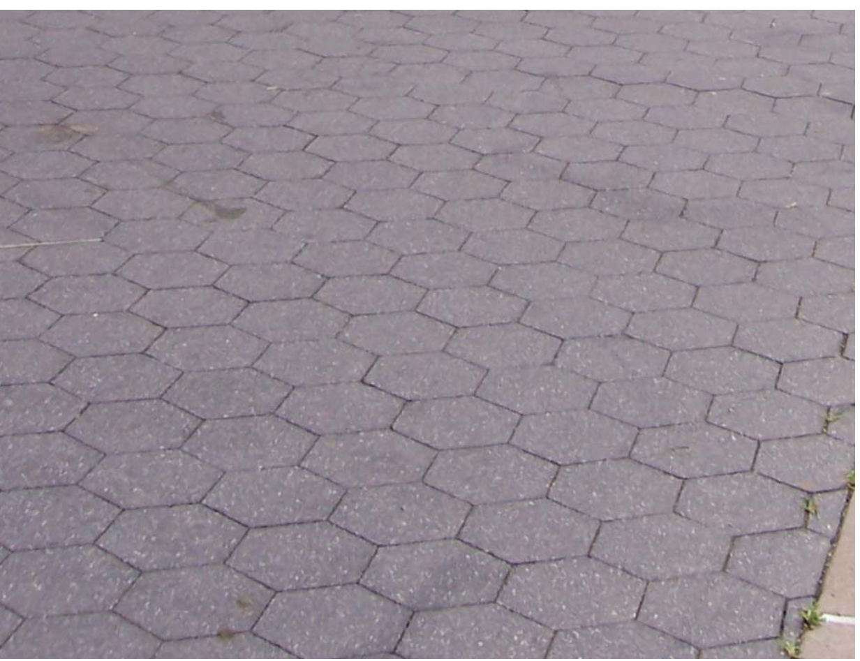
DPR STANDARD ASPHALT HEX PAVERS BY HANOVER FINISH : MATRIX #12
