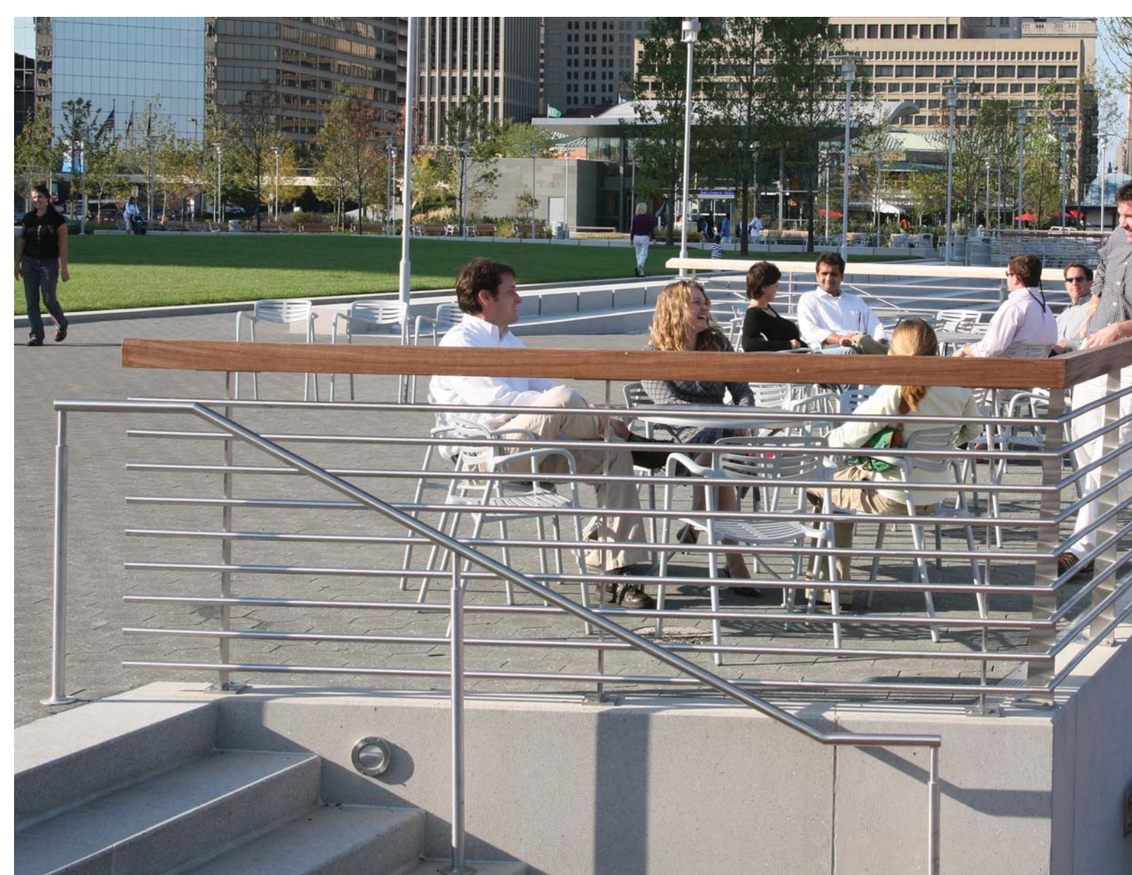
STAINLESS STEEL HANDRAIL
