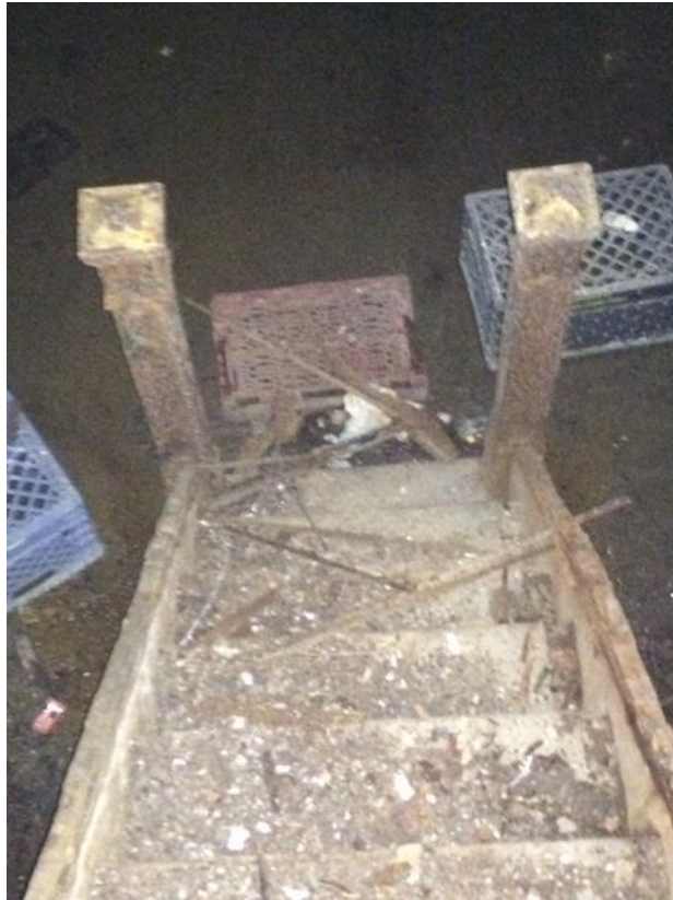
Photograph 3: View of the stairwell into the cellar level of the Lot 57 building, facing east.
