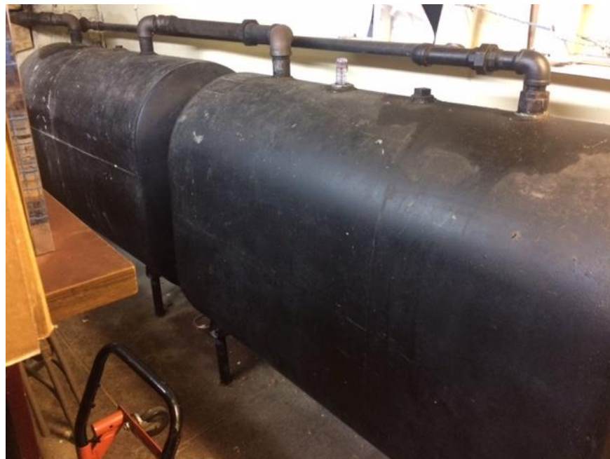
Photograph 14: View of the active 275-gallon aboveground storage tanks (ASTs) located in the cellar of the Lot 60 building, facing north.
