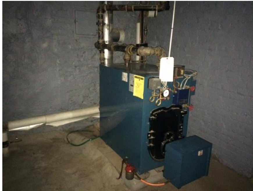
Photograph 13: View of the boiler room in the cellar of the Lot 60 building, facing east.
