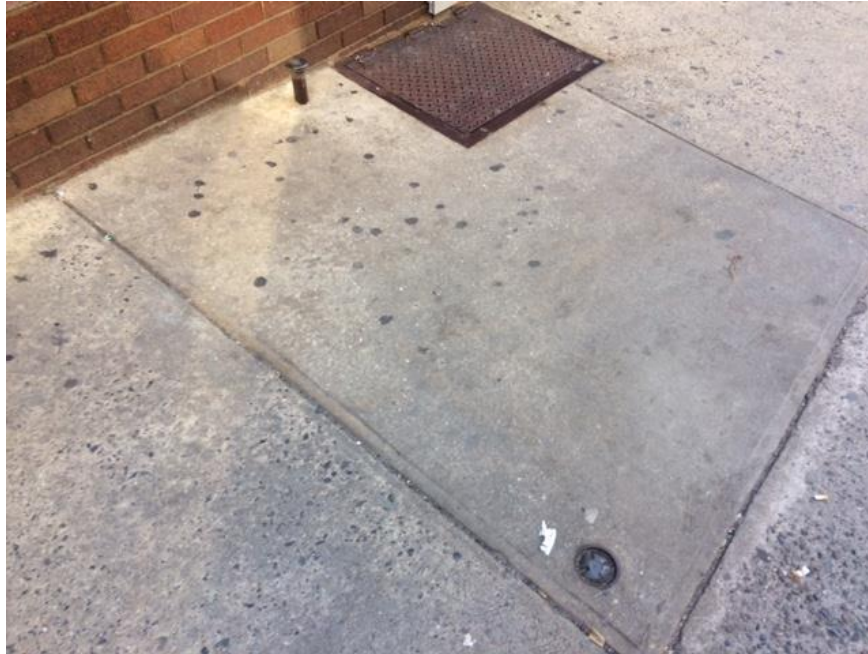
Photograph 11: View of the fuel oil fill port and vent pipe located on the sidewalk adjacent to the Lot 60 building, facing southwest.
