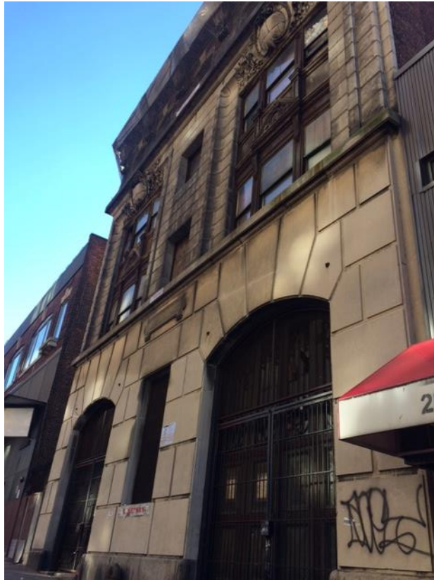
Photograph 1: View of Block 1243, Lot 57, facing southwest.
