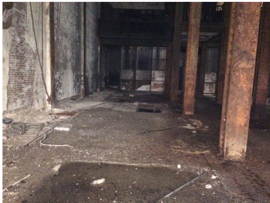
Photograph 2: View of the first floor of the Lot 57 building, facing south.
