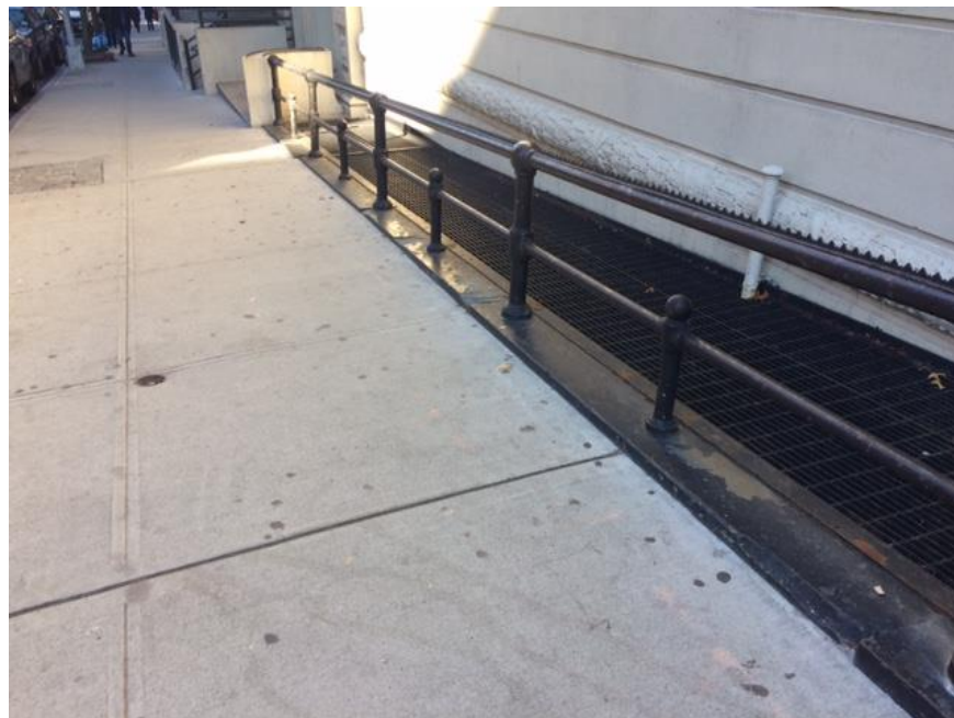
Photograph 20: View of vent and fill port located in front of a southern adjoining property, facing south.
