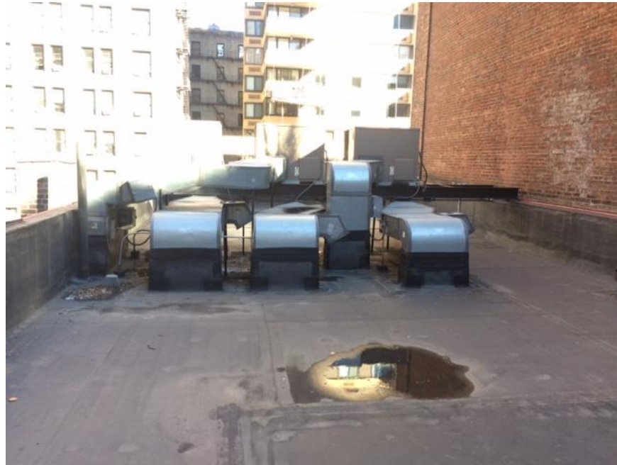
Photograph 9: View of the heating, ventilation, and air conditioning (HVAC) equipment on the roof of the Lot 59 building, facing north.
