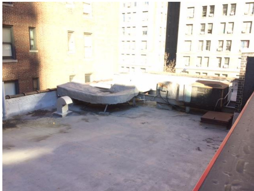
Photograph 18: View of HVAC equipment on the roof of the Lot 59 building, facing northwest.
