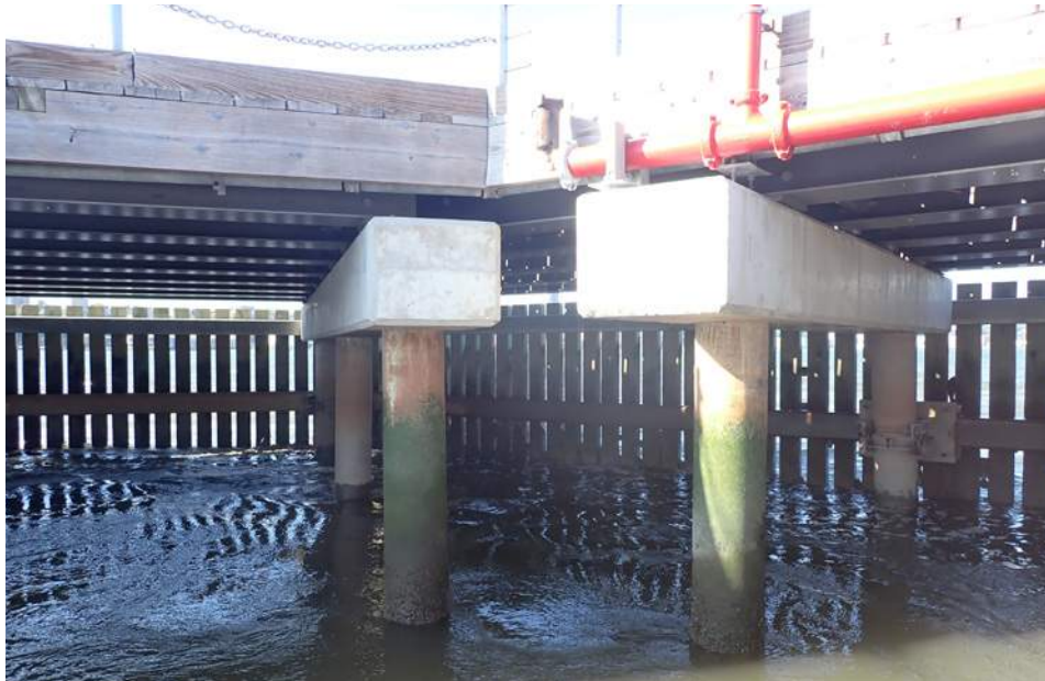
Steel Piles & Concrete Pile Caps
