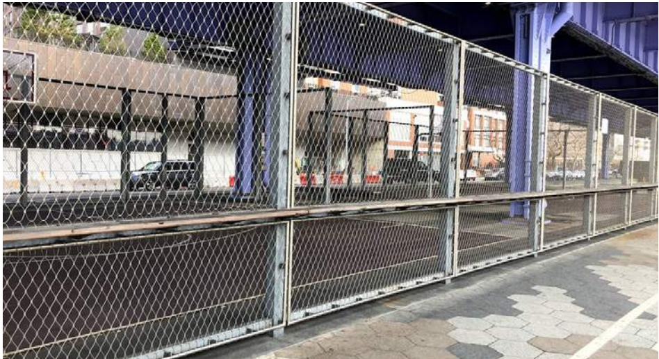
East River Waterfront Basketball Courts Stainless Steel Rope with Stainless Steel Tube Frames
