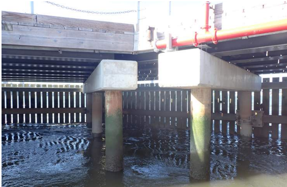
Steel Piles & Concrete Pile Caps
