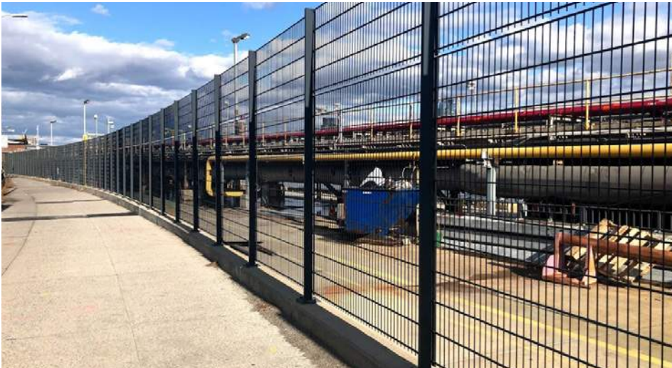
Con Ed Area Along East River Steel with Black Powder Coat Finish
