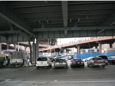
Parking under the FDR
