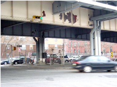
FDR existing conditions
