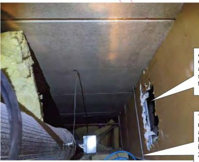
Above the ceiling, the underside of the concrete slab is visible. In addition, there are holes in the sides of the ceiling soffit leading to the outside building walls.
