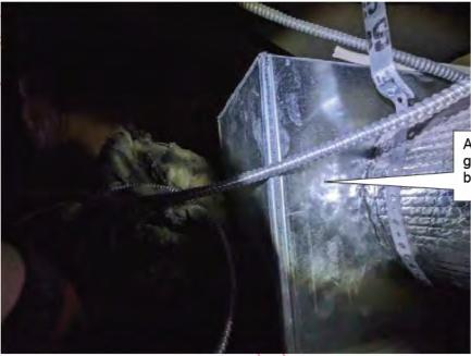
Above the air conditioning grills are sheet metal duct boxes.
