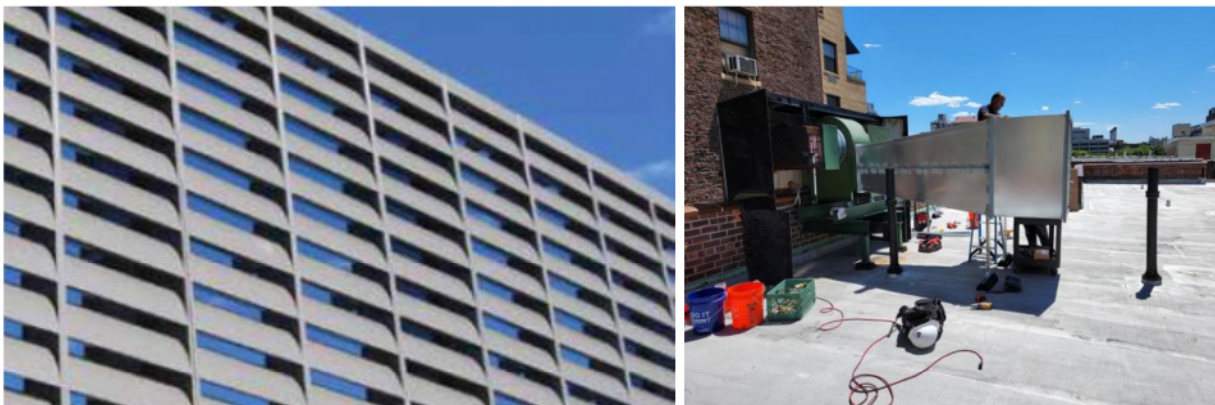
Figure 12 – (Left) photo of an acoustical louver system from IAC; (Right) Photo of a Noise Attenuator on a side-mounted grease exhaust system
