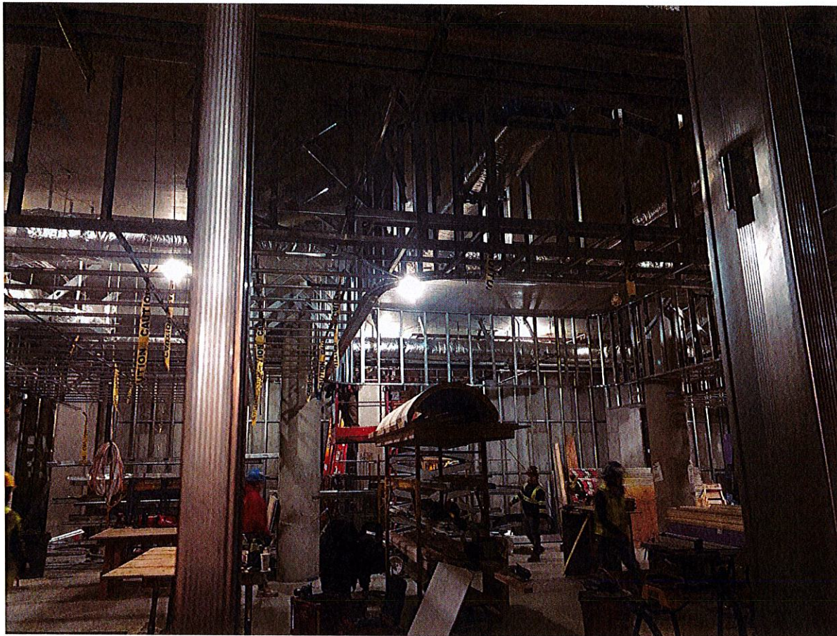
Cellar Level Bar/Restaurant Framing - 2.22.22
