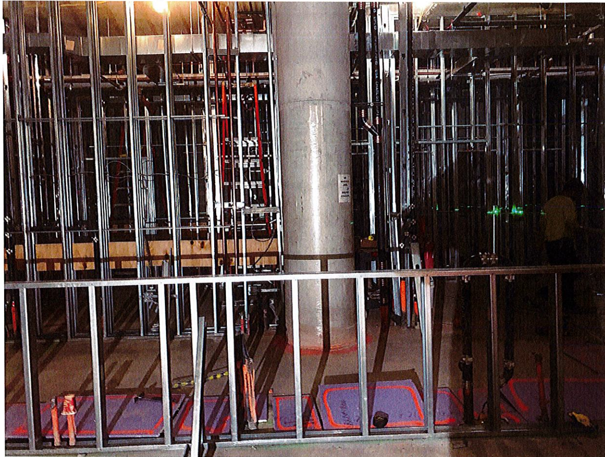
Sub Cellar Bar Area Framing
