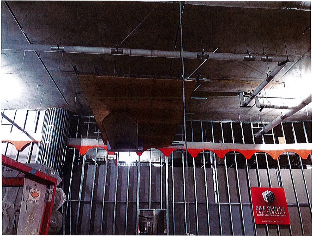
Ground Level – Lobby / Bar Area Wall & Ceiling Framing 2.22.22
