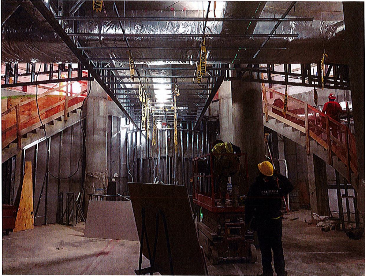
Cellar Level Grand Stair Bar Area Framing - 2.22.22
