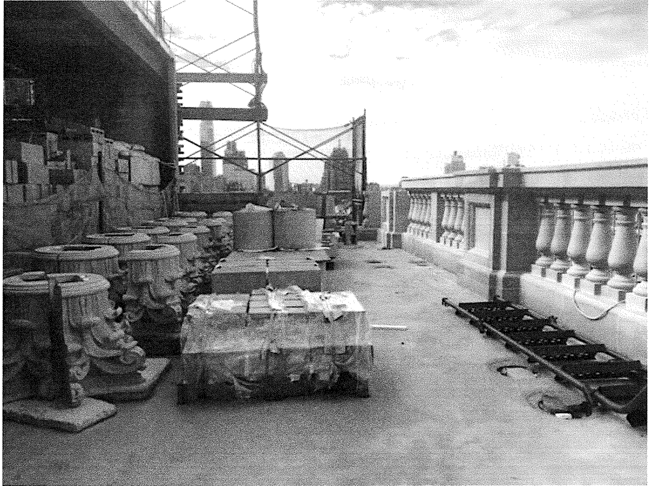
Location: Parapet, 14 th Floor
