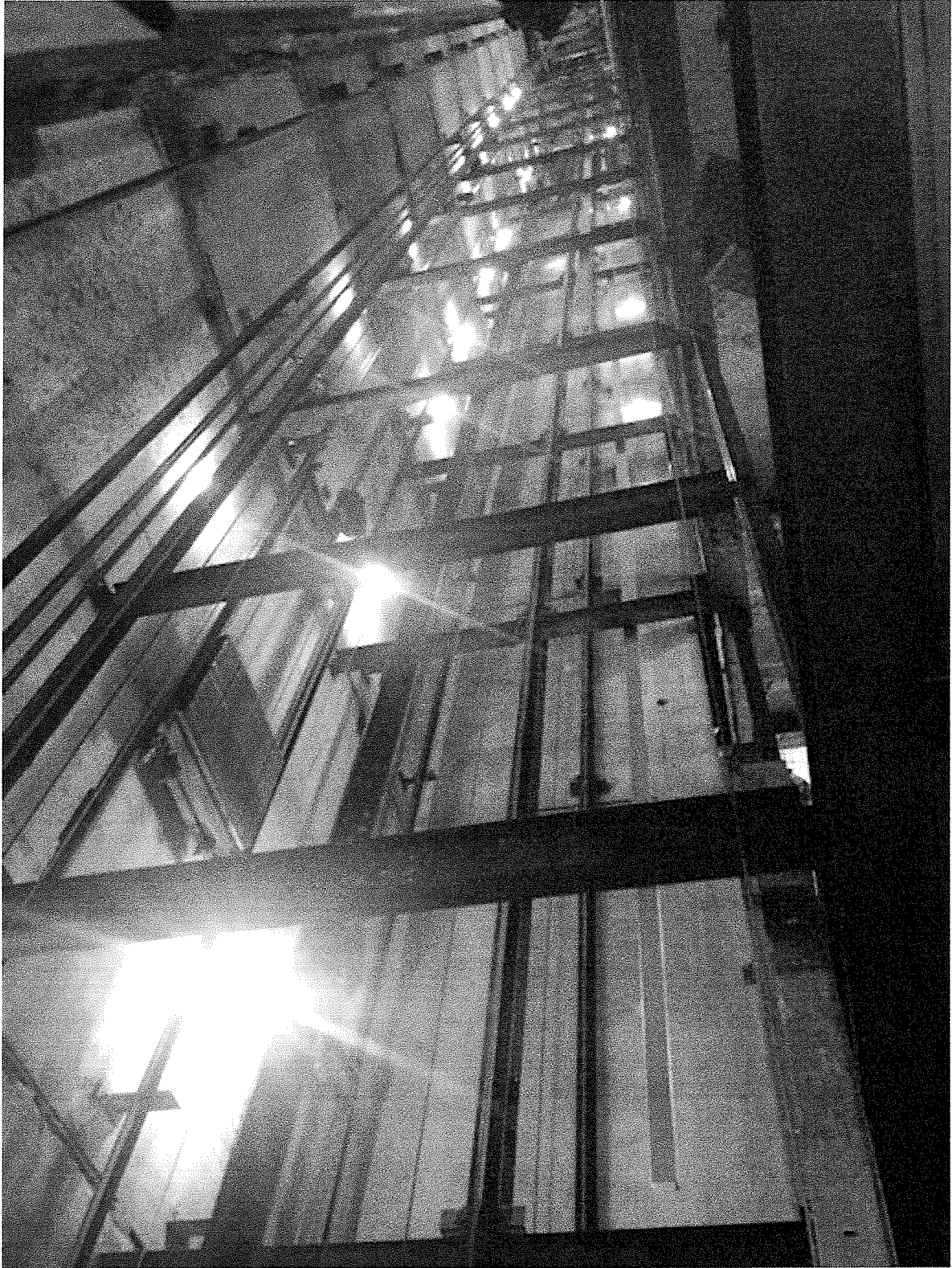
Location: Elevator Shaft
