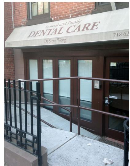
Figure 34: Example of Permanent Ramps
