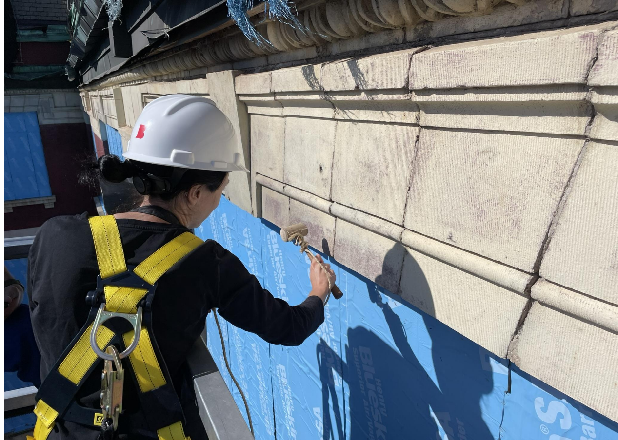
SURVEYING CONDITIONS FROM AN AERIAL LIFT, SOUNDING TERRA COTTA UNITS WITH A Mallet TO DETERMINE CONDITION
