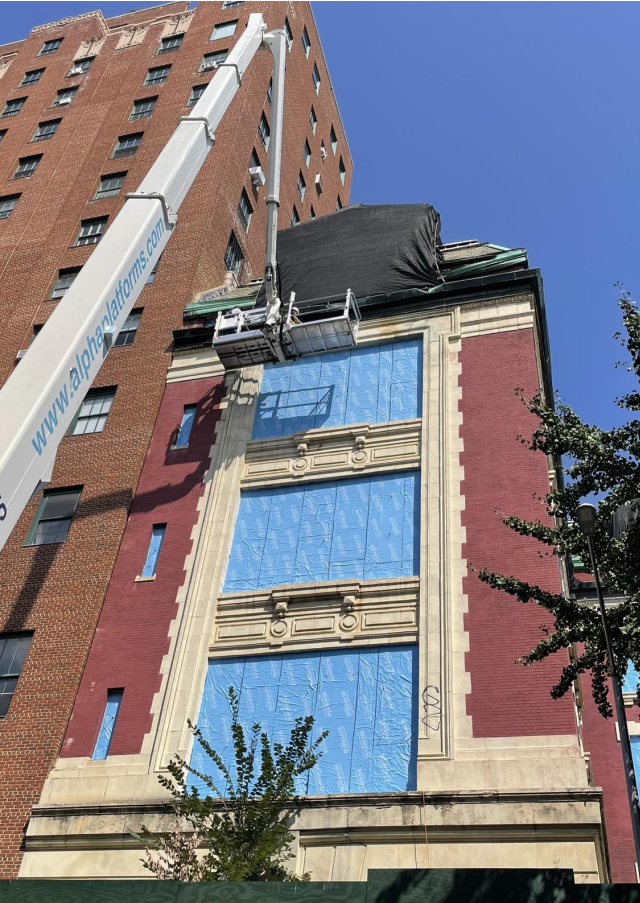
SURVEYING CONDITIONS FROM AN AERIAL LIFT, SOUNDING TERRA COTTA UNITS WITH A Mallet TO DETERMINE CONDITION
