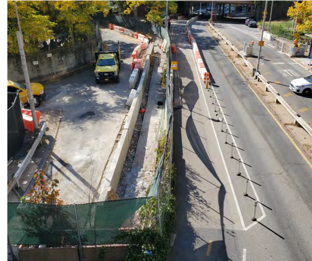
Pinch Point Sidewalk Construction, Fall 2024
