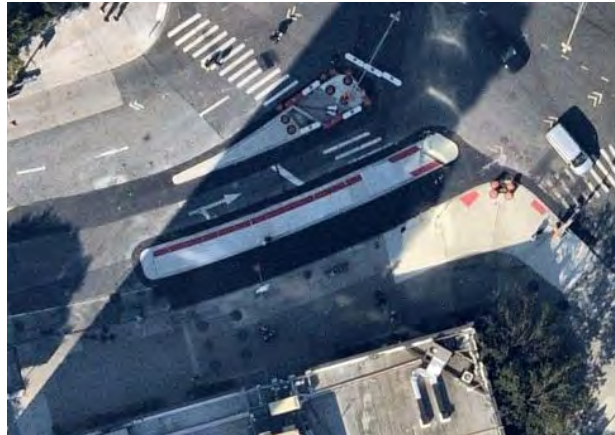
Bus Stop Island Construction
