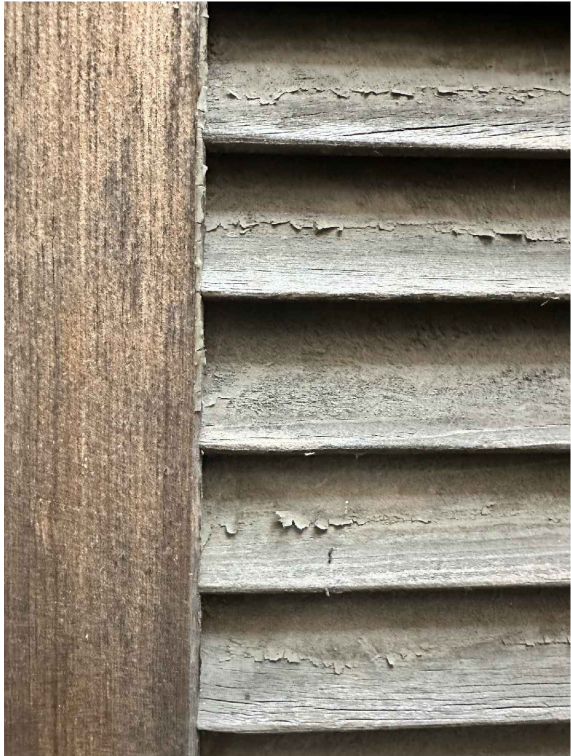
WOOD SHUTTERS THAT ARE DETERIORATED TO BE REPAIRED TO MATCH EXISTING.
