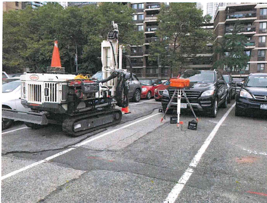
Photo 2: AARCO installing sub-slab vapor probe at Void 5 (facing north)
