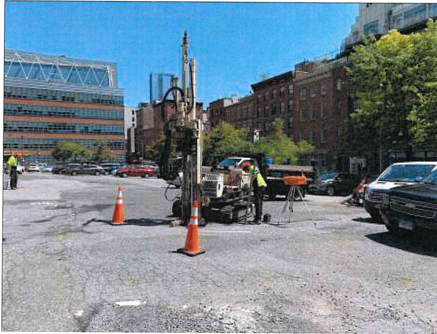
Photo 3: AARCO drilling boring SB16 (facing east).
