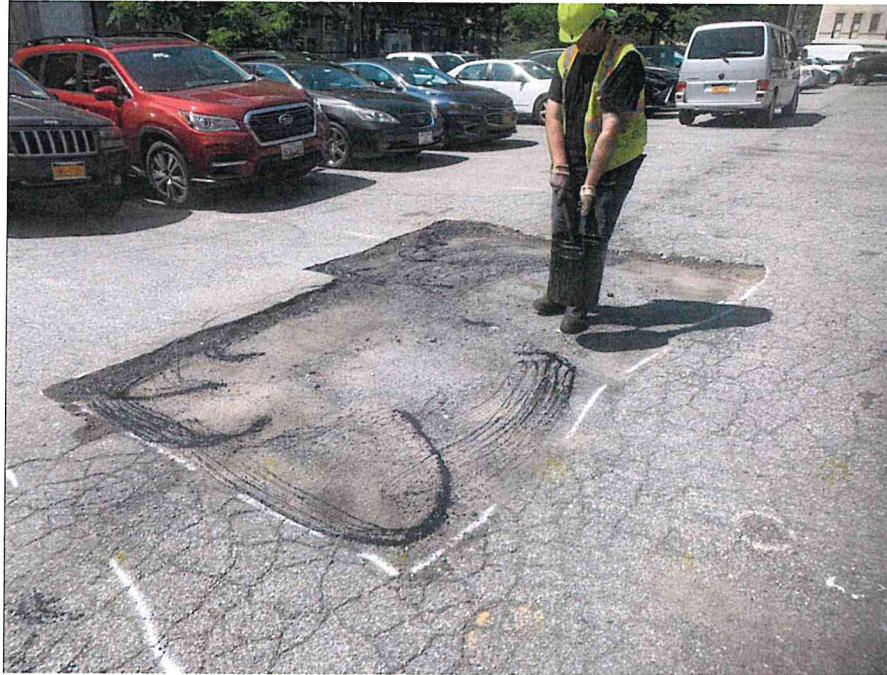
Photo 1: View of cut edges in the existing asphalt and placement of AC-5 (facing project southwest)
