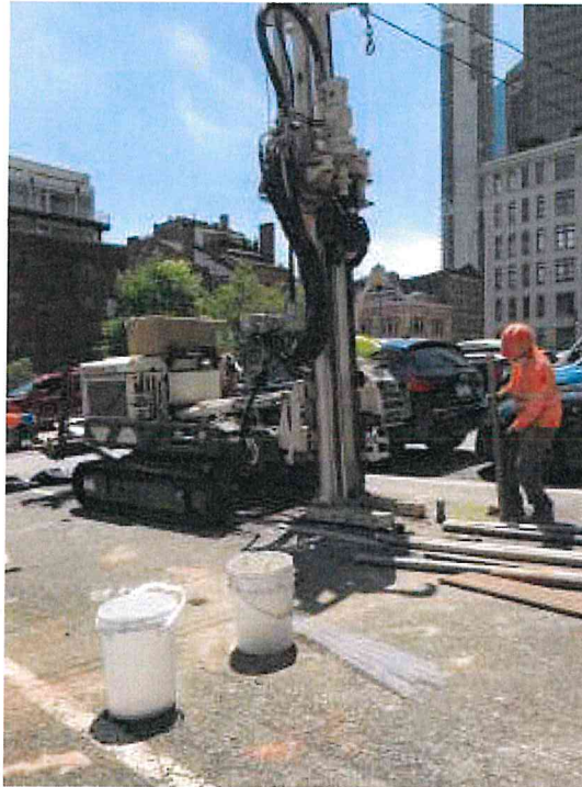
Photo 1: AARCO advancing soil boring SB4W1 (facing southwest)
