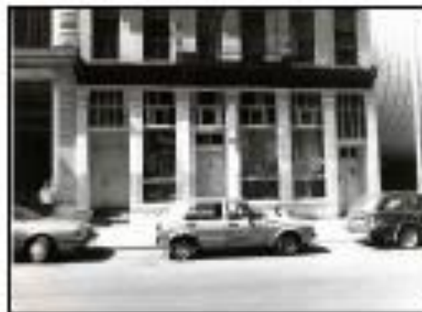
LPC DESIGNATION PHOTO OF GROUND FLOOR
