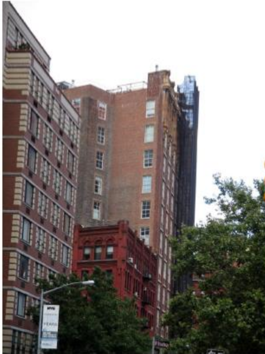
1) VIEW FROM SE CORNER OF CHAMBERS & WEST BROADWAY
