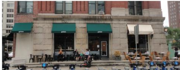
FRANKLIN STREET | EXISTING STOREFRONT
