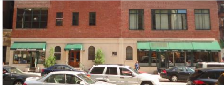
VARICK STREET | EXISTING STOREFRONT
