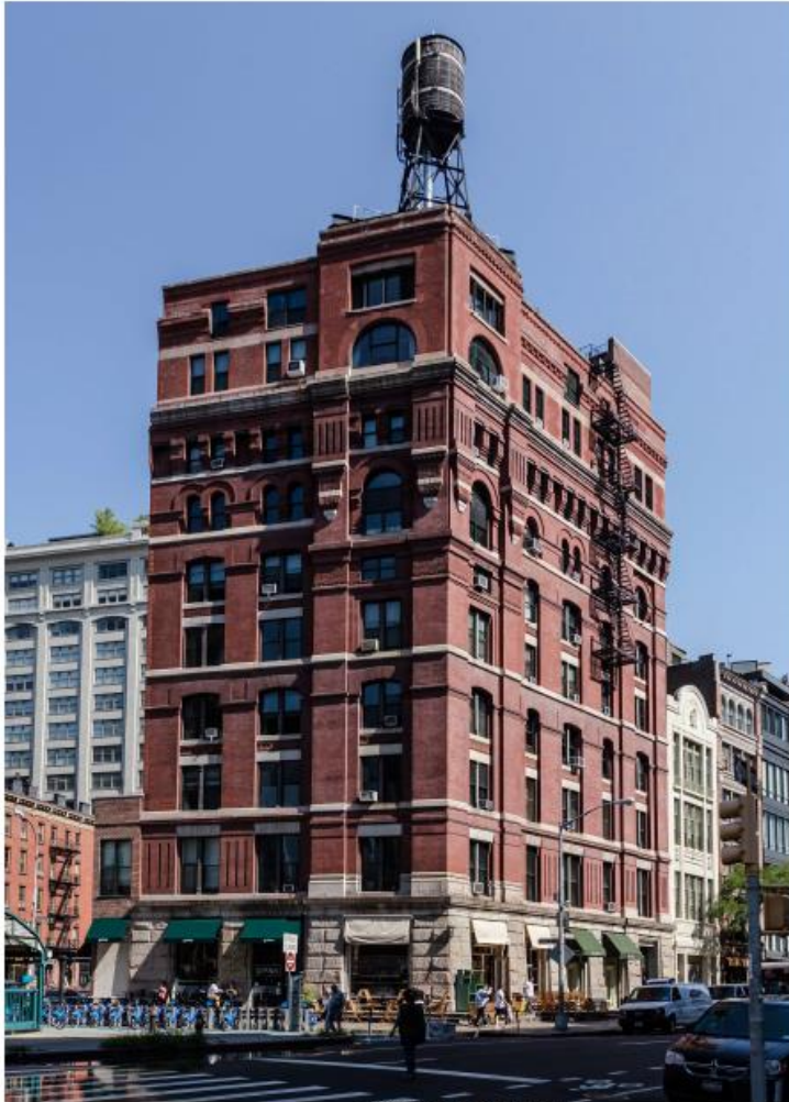
6 VARICK STREET | SOUTHEAST CORNER
