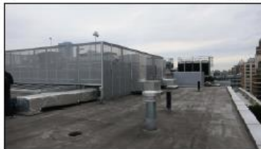
30 EXISTING CONDITIONS AT PENTHOUSE ROOF, LOOKING NORTHEAST NOT TO SCALE
