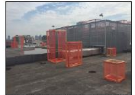
28 MOCK-UPS AT PENTHOUSE ROOF, LOOKING NORTHEAST NOT TO SCALE
