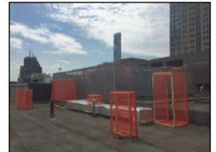
31 MOCK-UPS AT PENTHOUSE ROOF, LOOKING SOUTHEAST NOT TO SCALE
