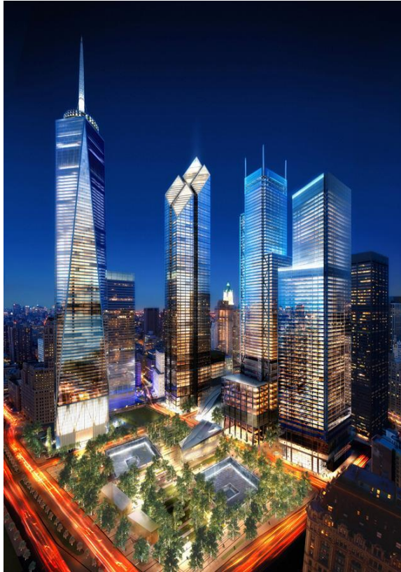
WTC Construction Site 7 WTC – Moody's Pedestrian Safety Managers
