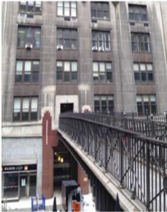
EXISTING FACADE AT TRINITY PLACE
