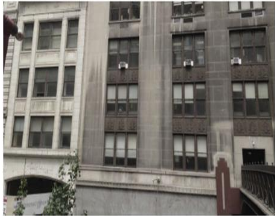
EXISTING SPLIT BUILDING
