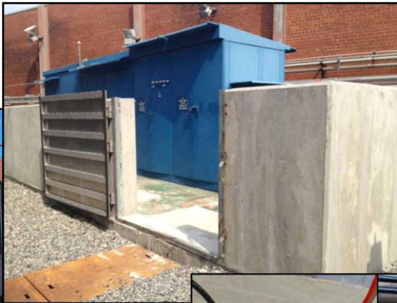
E. 13 th St. S/S – Concrete Moat & Door
