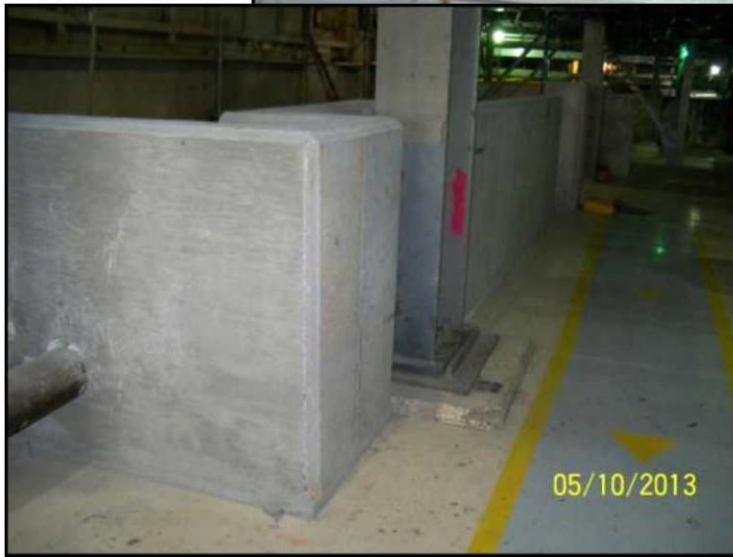
East River – Internal Concrete Moats
