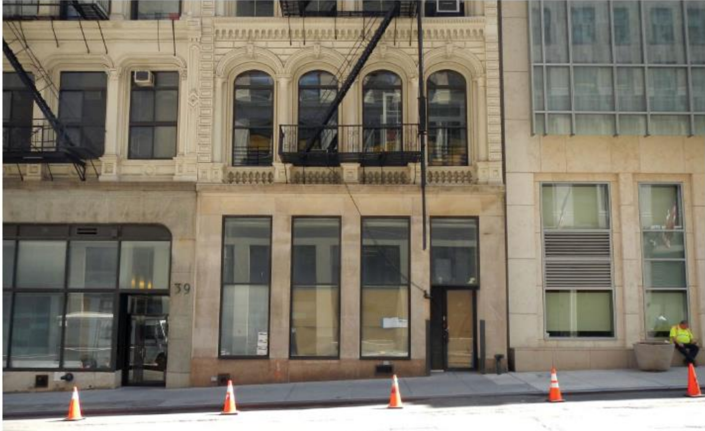
VIEW OF EXISTING STOREFRONT ON WORTH STREET
