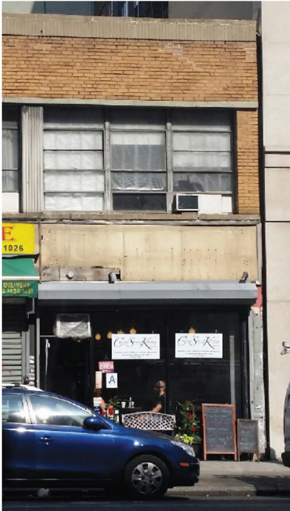
① PHOTO OF CURRENT AREA OF WORK NTS
