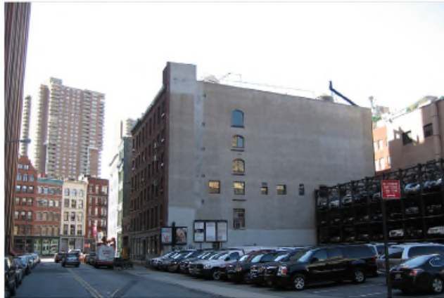
VIEW OF EAST FACADE
