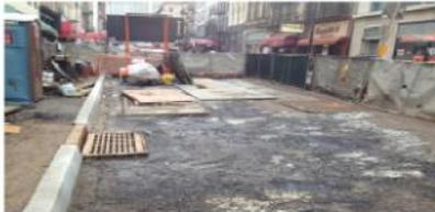
Road Base and Granite Curb have been installed in the Northwest area of Chambers Street and West Broadway
