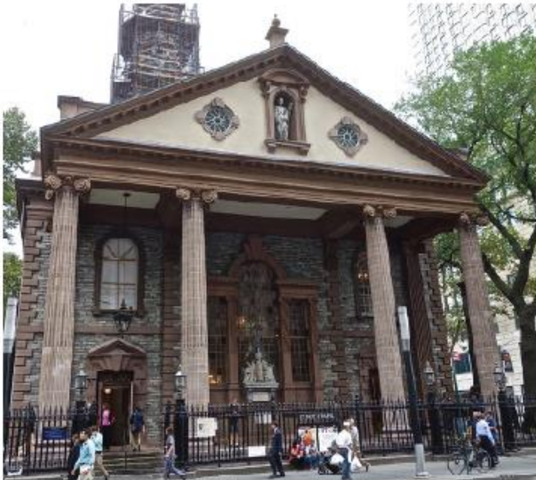
1. East elevation of St. Paul's Chapel after 2014 restoration and prior to August 2015 removal of sculpture from the site by the contractor
