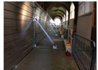
Flood Wall Installation on Vesey Street
