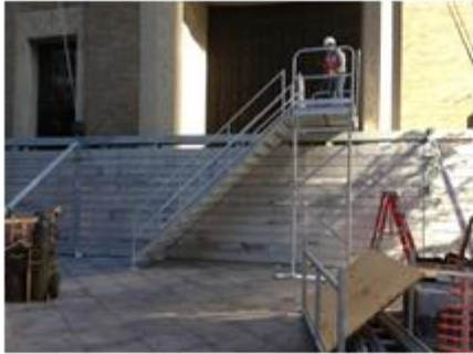
Egress Stair & Flood Wall Installation on West Street
