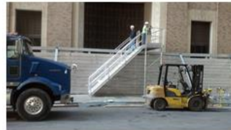
Egress Stair & Flood Wall Installation on Washington Street
