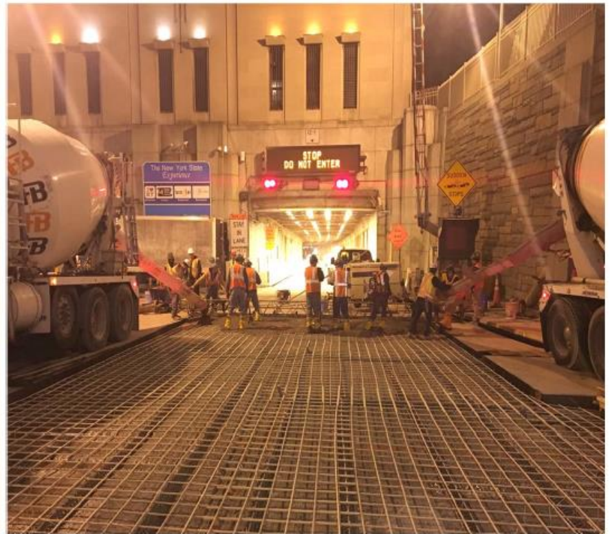
HLC Manhattan Plaza work during West Tube closure
