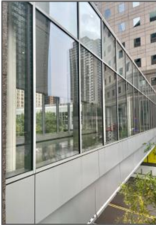
Liberty St. Bridge
